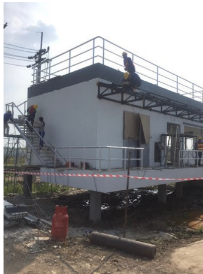
Photo 2: Welding and gas cutting without face masks or shielding for
