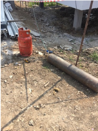
Photo 1: Unrestrained gas cylinders for gas cutting.
