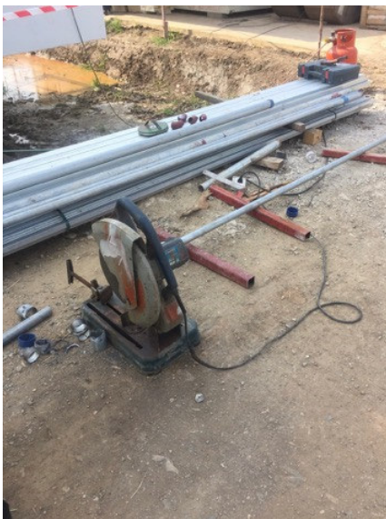
Photo 3: Electrical cables, sockets and tools on open ground.
