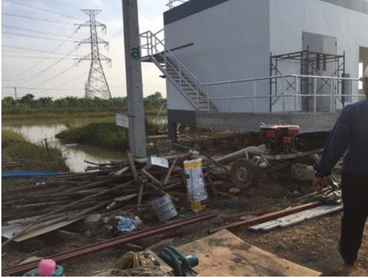
Photo 4: Waste pile trip and fall hazard. Power tools on open ground.
