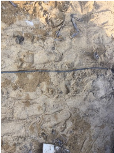
Photo 6: Electrical cable running over open ground.
