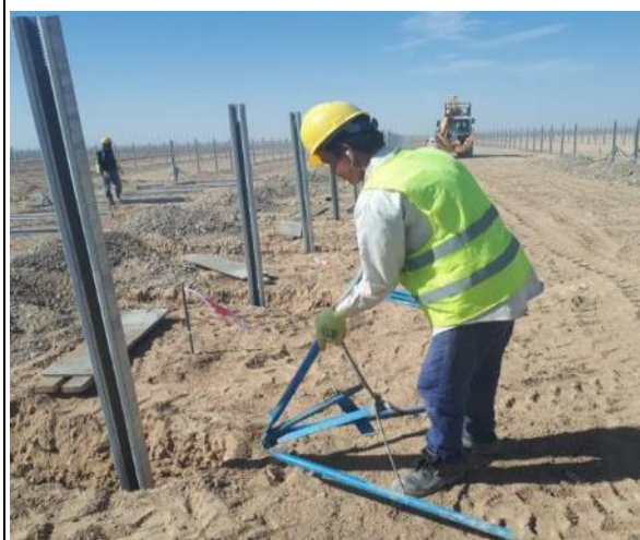
Figure 3: Project site during construction
