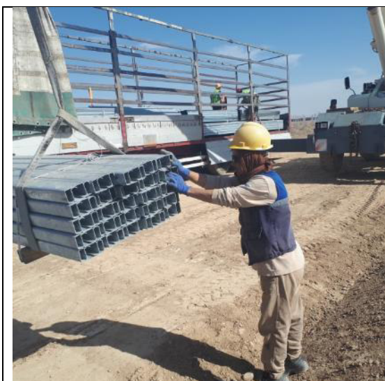
Figure 18: Workers with PPE
