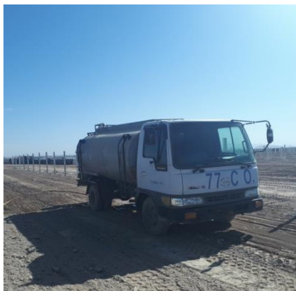
Figure 34: Water sprinkling at the project site
