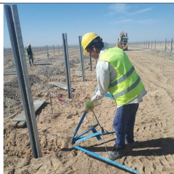
Figure 19: Workers with PPE
