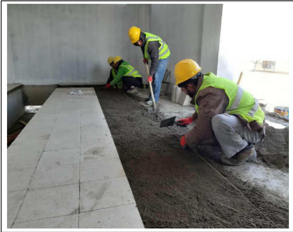
Transformer buildings floor tiles are in progress.
