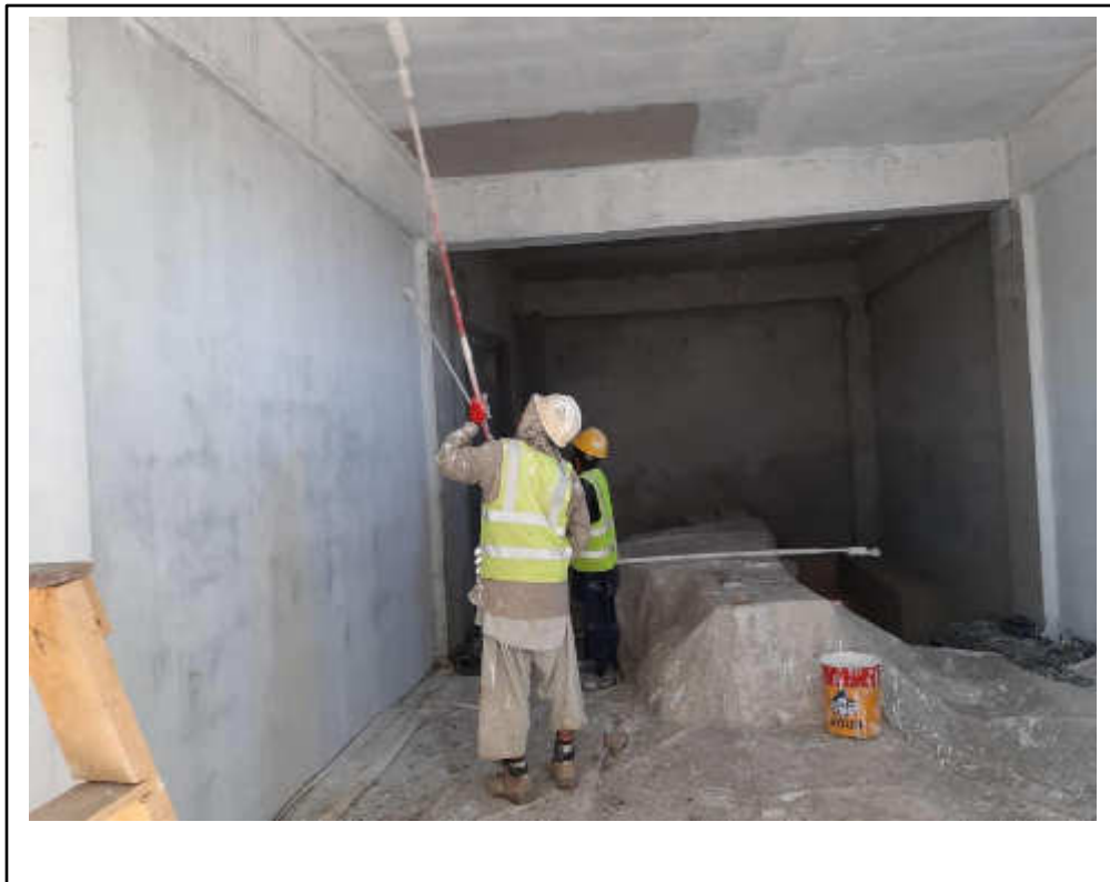
Distribution center building paint in progress
