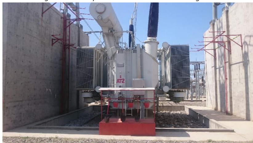
Fig. 12. Auto-transformer equipped with automatic fire-extinguishers at Sughd SS
