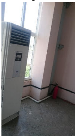
Fig. 15. Telecom and protections computer rooms that count with electronic equipment were refrigerated to avoid over-heating at Regar SS.
