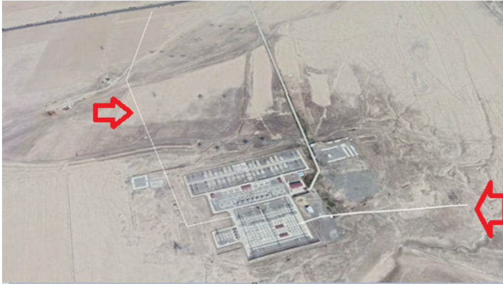
Figure 5. Conductors of route option 3 for the new stretches of the OHTL (red arrows).
