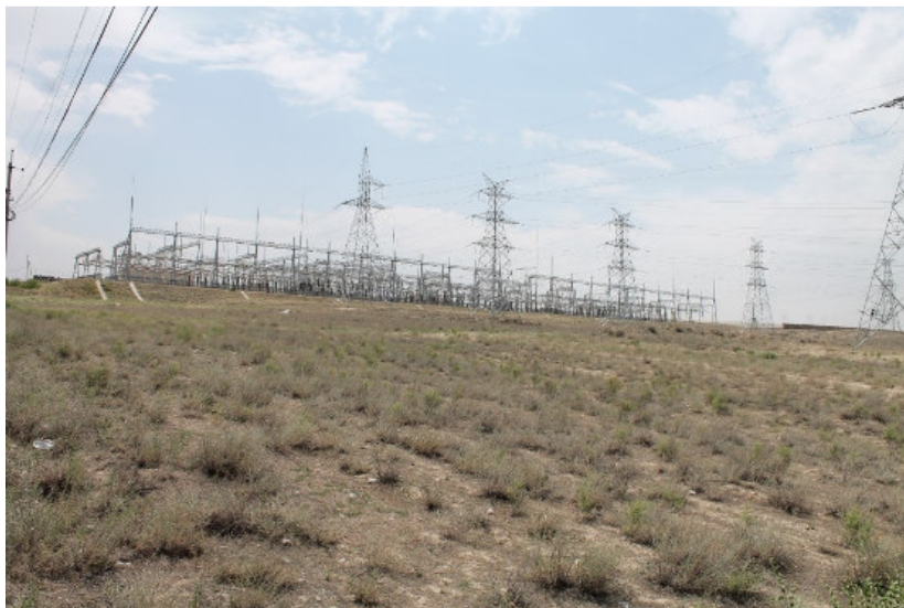
Figure 6. Land around the Sughd Substation, non-arable.
