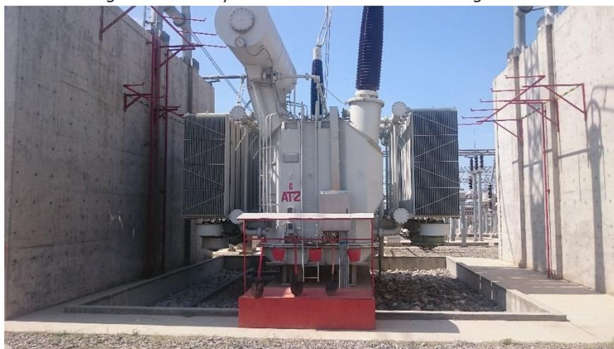
Fig. 13. Auto-transformer equipped with automatic fire-extinguishers at Sughd SS
