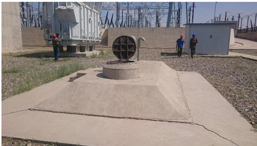
Fig. 14. Oil collection tank that is conducted leaked oil from the auto-transformers via pipes at Sughd SS
