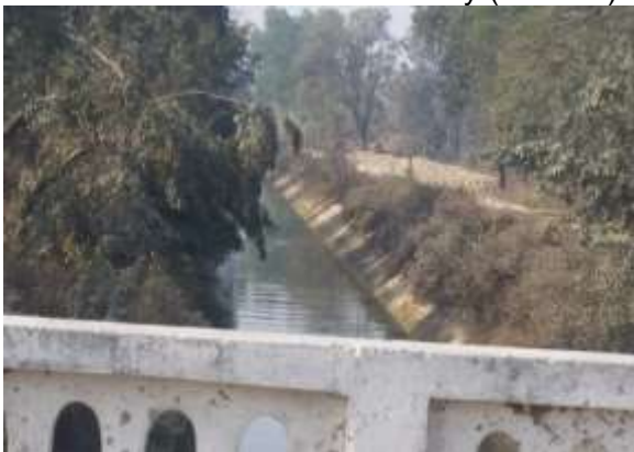
Photo 11: Canal crossing at Ch. 84+700
