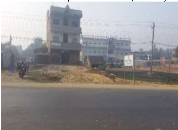
Photo 5: School alongside the road (48+200)
