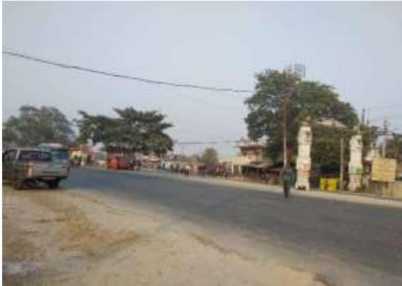
Photo 1: Start point (00+000), Kanchanpur
