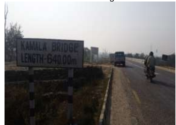
Photo 12: End point of Road (87+000)
