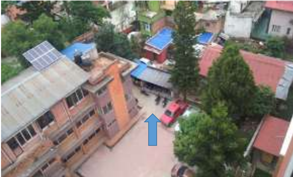
Photo 3: Existing parking area and staff quarter of the Directorate
