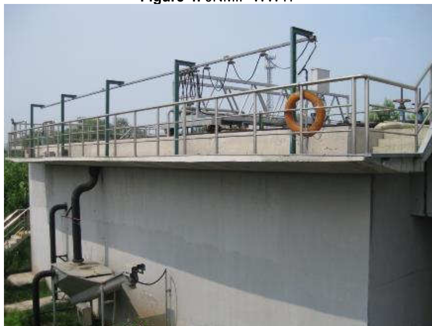
(i) Screen room and aerated grit chamber
