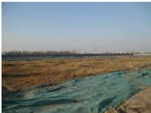
(i) Construction site is covered for dust control
