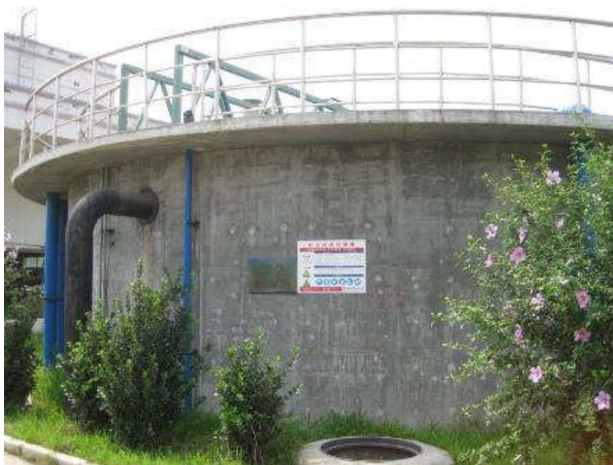
(iii) Sludge concentration tank
