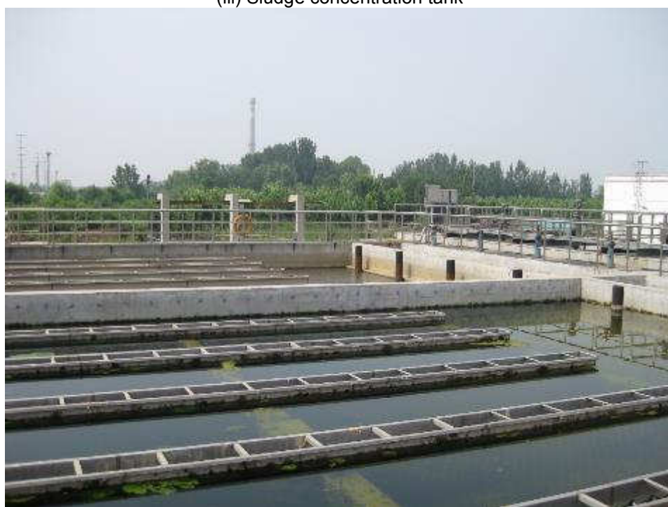
(iv) Flocculation precipitation and sand filter tanks
