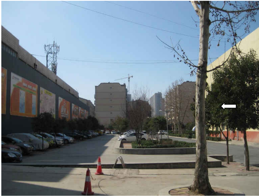
Figure 5: Cooling tower location in Dongxin TPP layout
