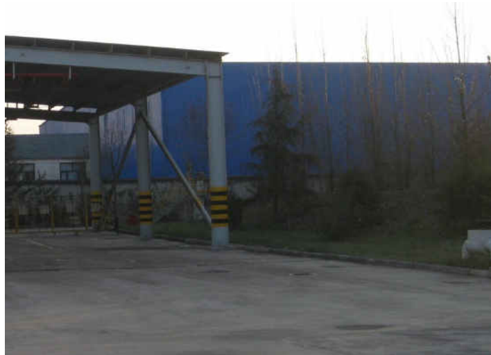
Figure 17: Closed coal storage room, Zhangqiu TPP
