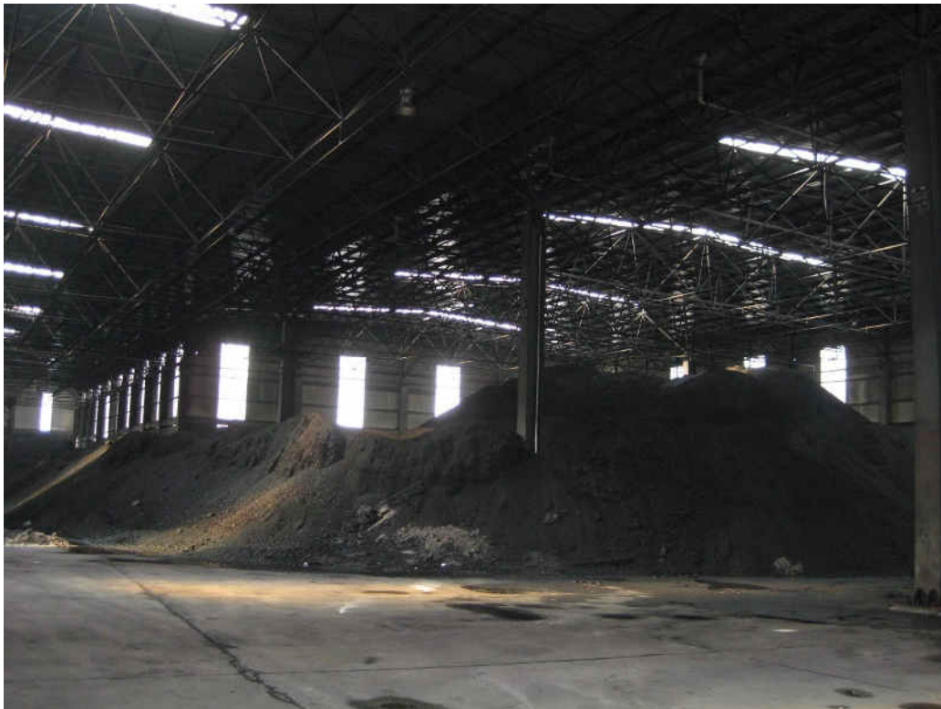
Figure 6: Coal storage room, Dongxin TPP
