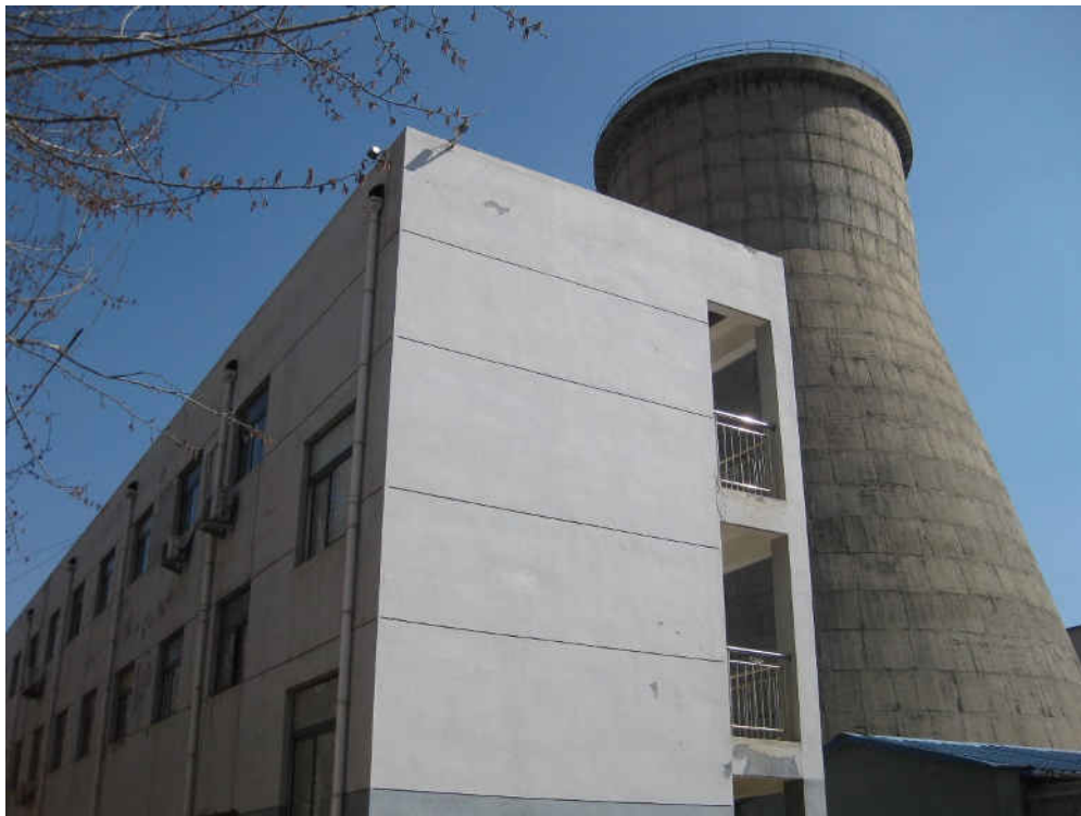
Figure 7: Dongxin TPP cooling tower and office building
