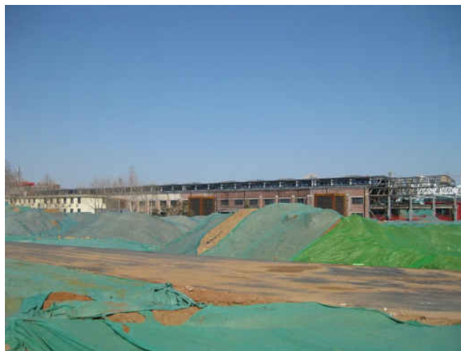
(iii) The whole area is under construction.
