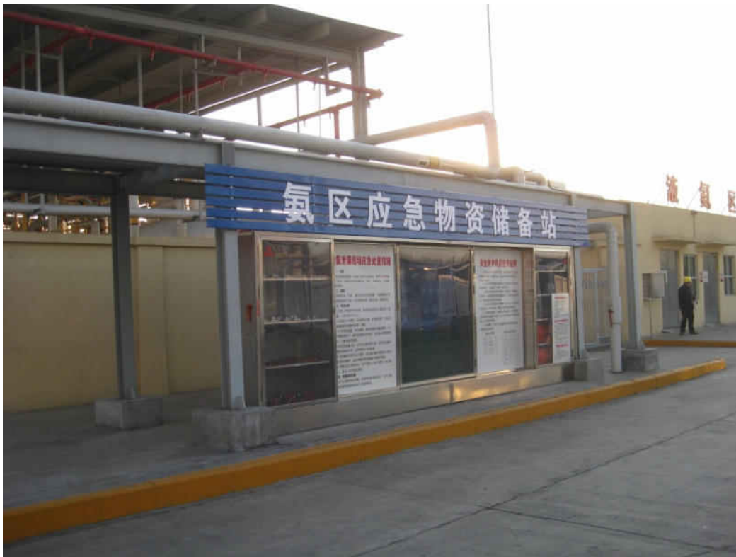
Figure 19: Zhangqiu TPP liquid ammonia storage area
