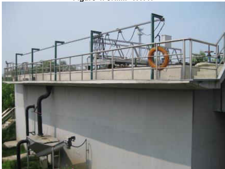
(i) Screen room and aerated grit chamber
