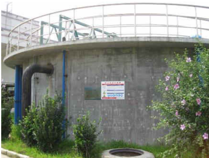
(iii) Sludge concentration tank
