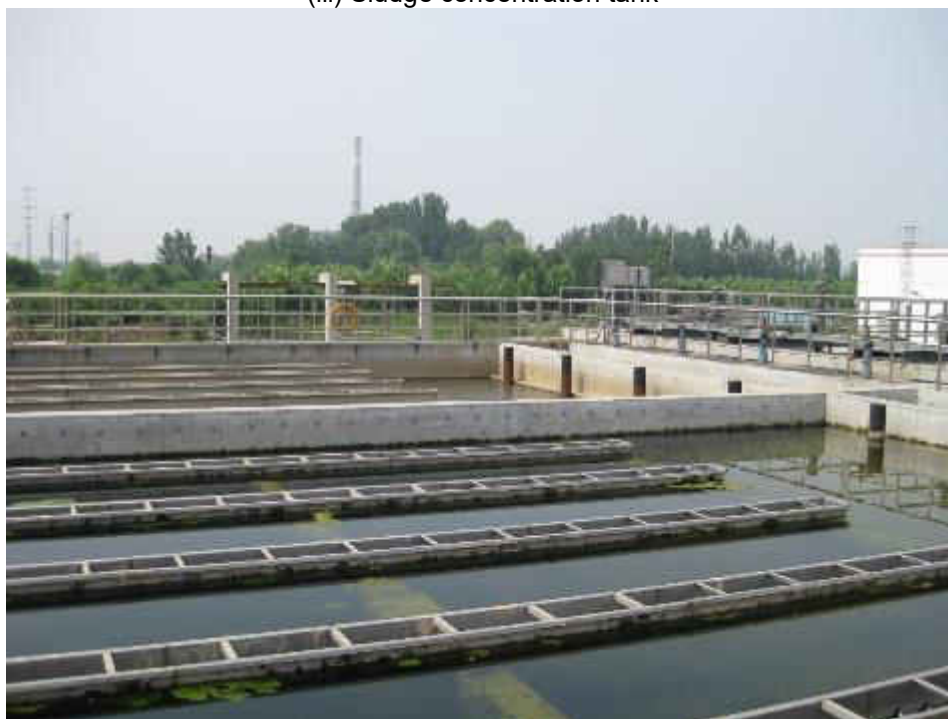
(iv) Flocculation precipitation and sand filter tanks
