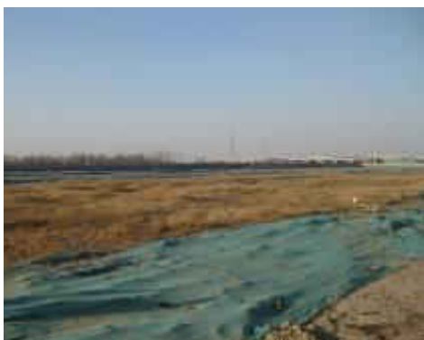
(i) Construction site is covered for and dust control
