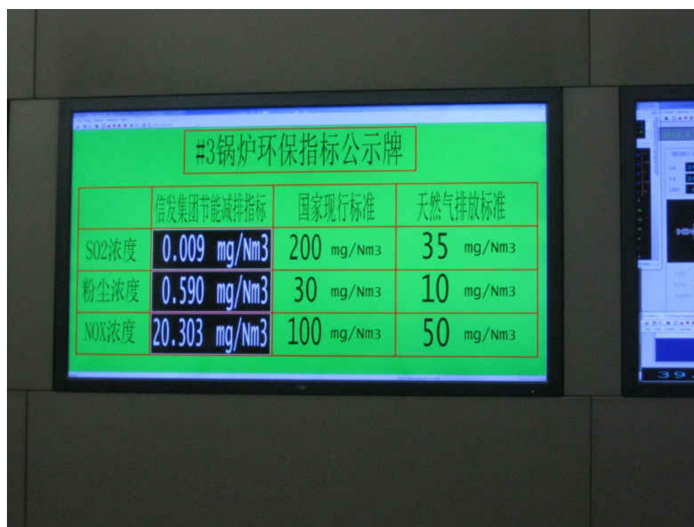
Figure 7: Xinyuan Power Plant real-time CEMS data
