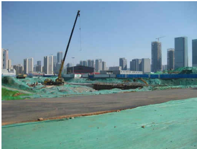
(ii) Construction site is covered for and dust control.
