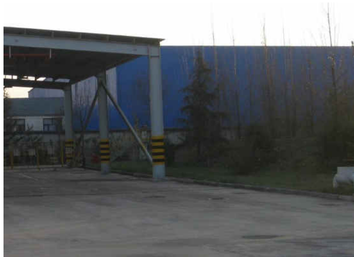
Figure 17: Closed coal storage room, Zhangqiu TPP
