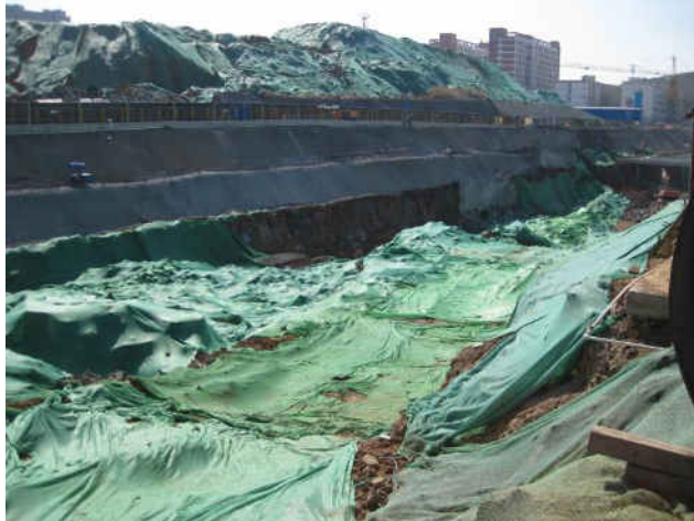
(i) Construction site is covered for and dust control
