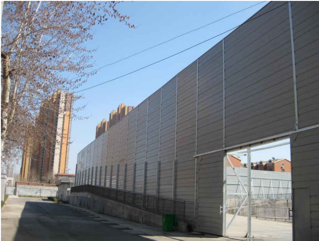
Figure 8: Dongxin TPP noise barrier
