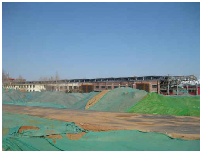
(iii) The whole area is under construction.
