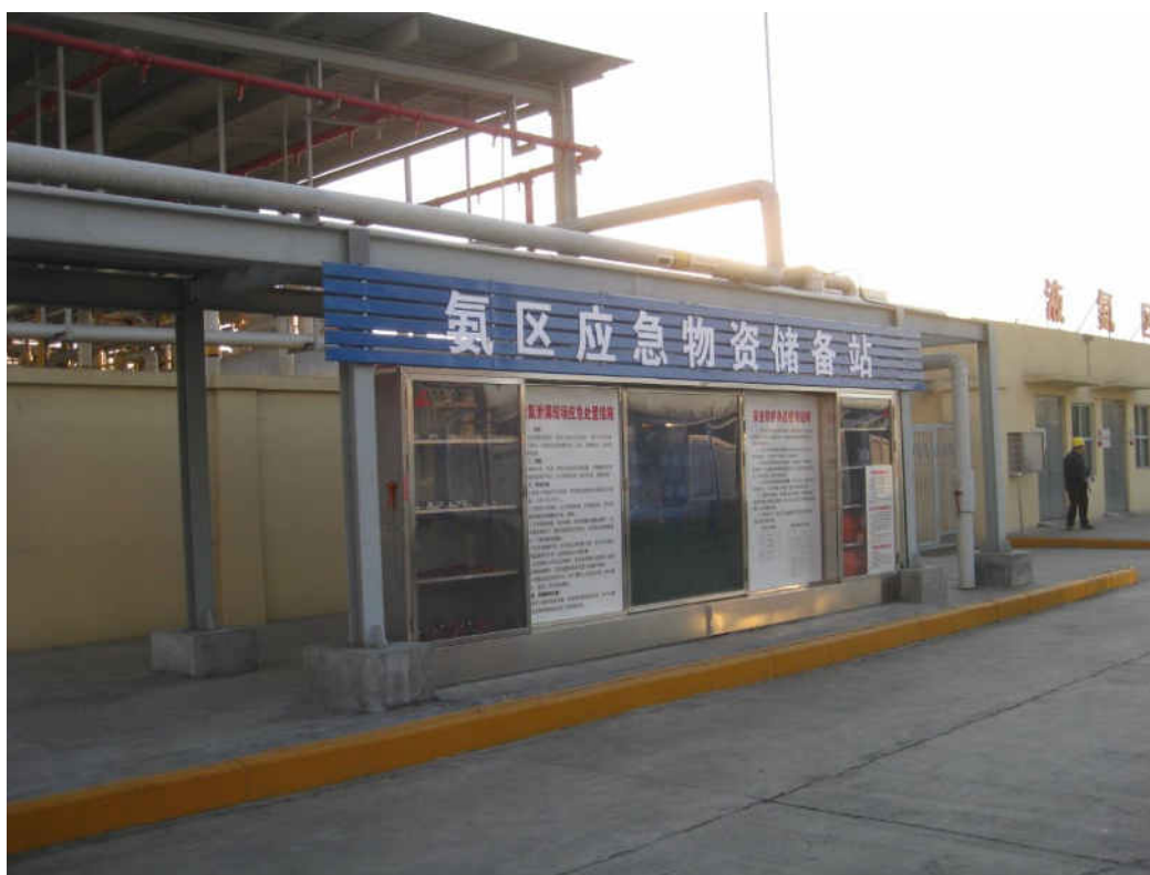
Figure 19: Zhangqiu TPP liquid ammonia storage area
