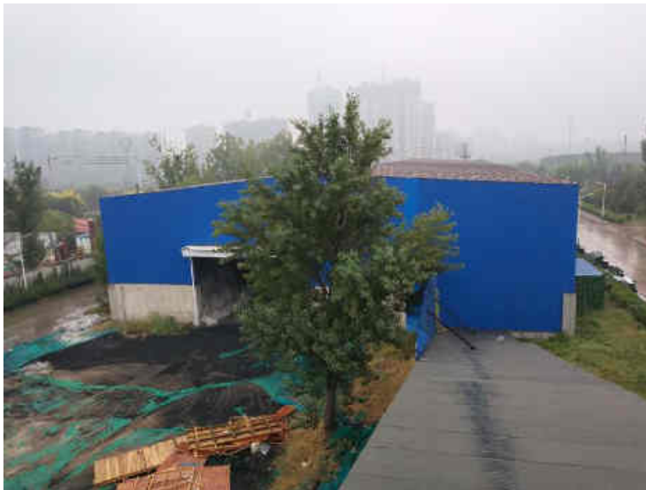
Figure 4: Closed Coal Storage Room
