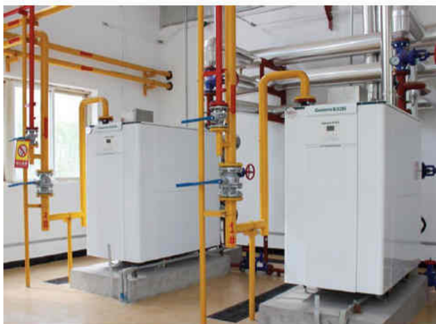
Figure III-8: Installation Instruction of Gas Modular Boiler
