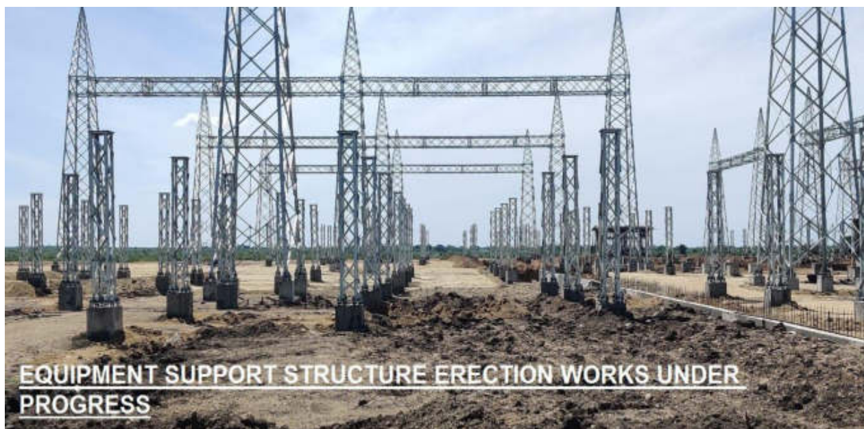
Image 2: Equipment support structure erection works under progress in Virudhunagar Substation
