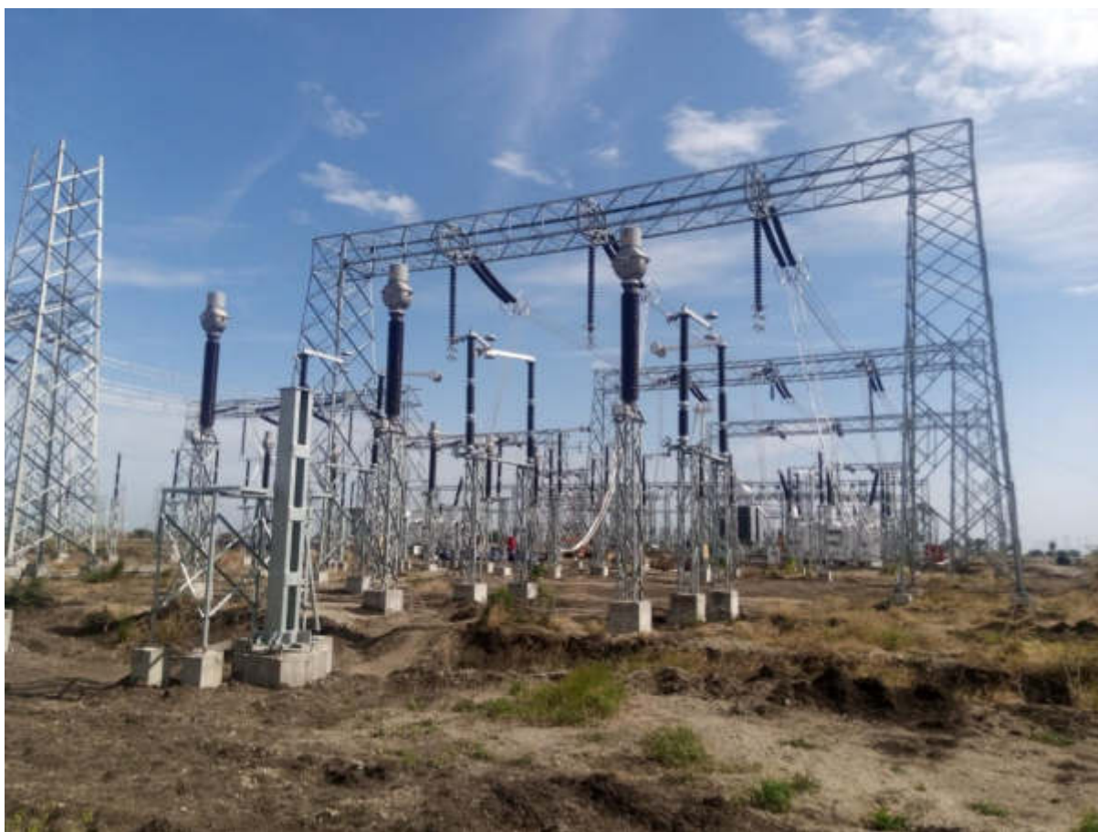
Image 6: 400 kV equipment installation work in Ottapidaram Substation
