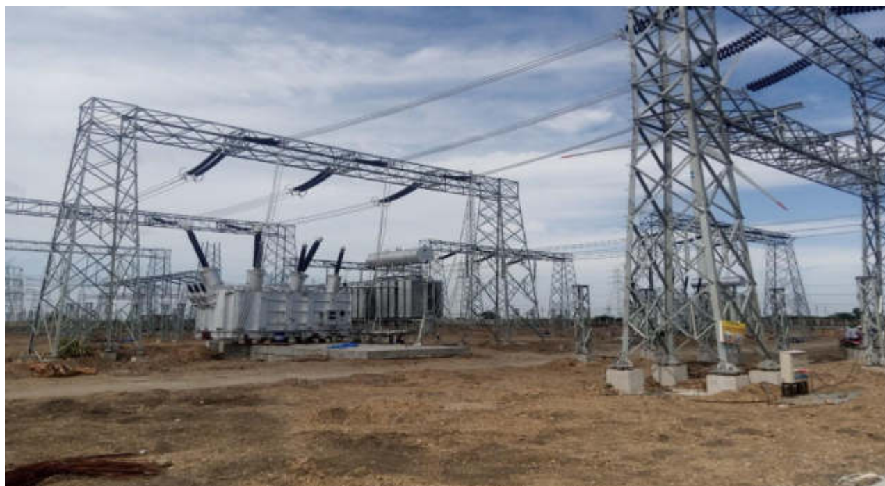
Image 4: Erection of 500 MVA Transformer in Ottapidaram Substation
