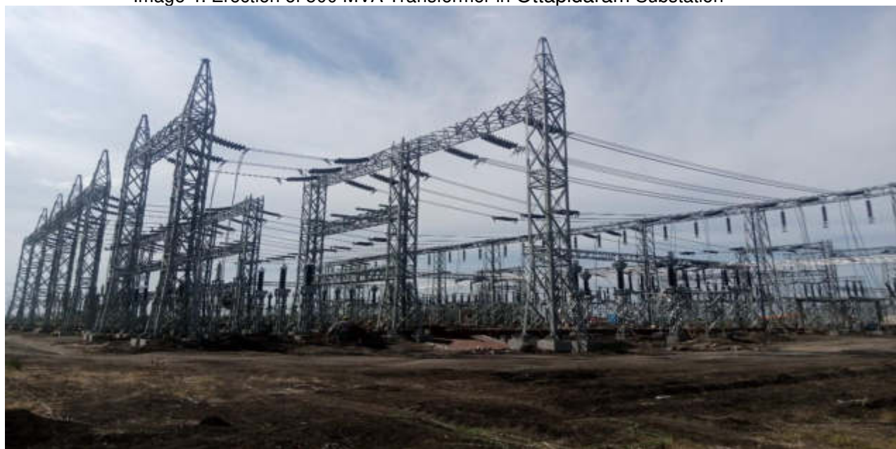
Image 5: 230 kV stringing & equipment installation work in Ottapidaram Substation
