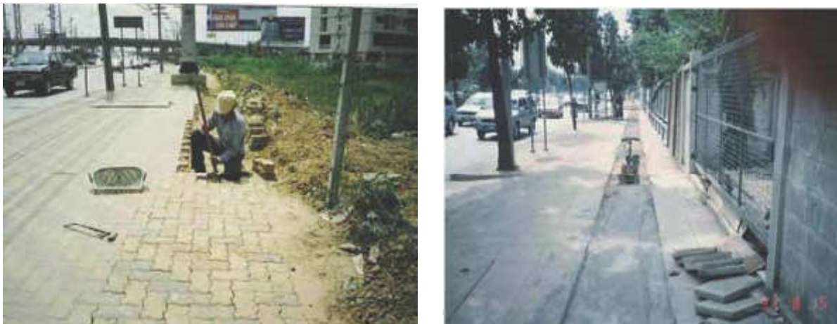
Figure 7.3.3 - 3 The maintenance of sidewalks at the end of construction phase
