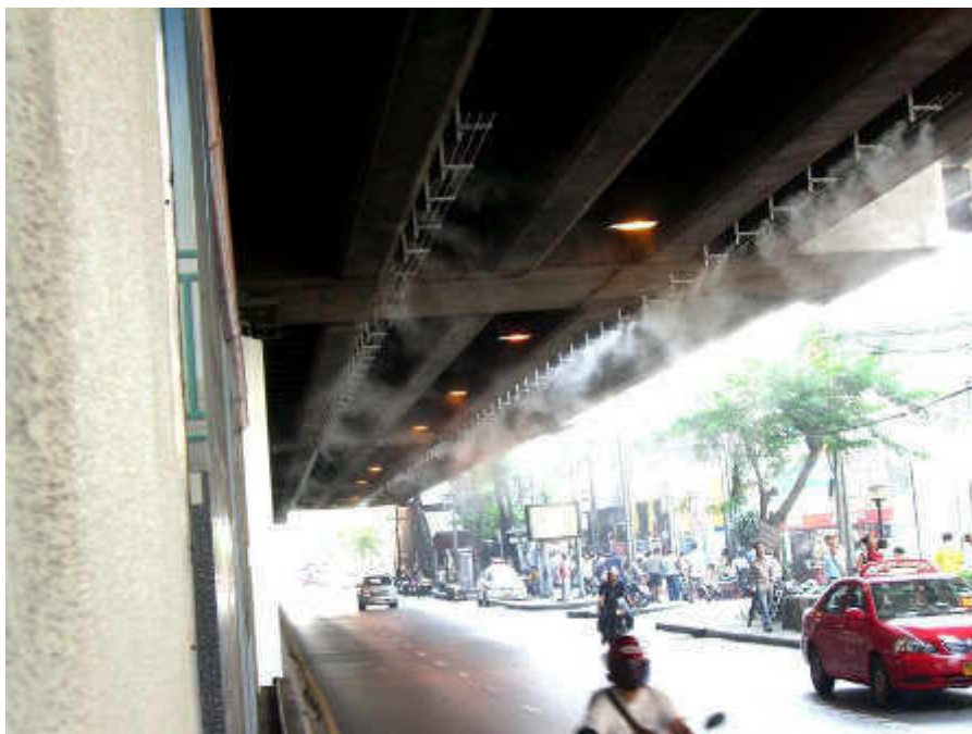
Figure 7.1.5 - 1 The example of spray nozzles installed under the MRT stations
