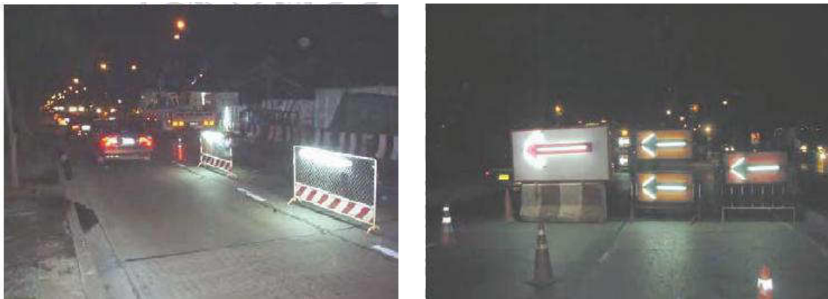
Figure 7.3.3 - 1 Example of information board, construction signs, and traffic signs during the construction phase
