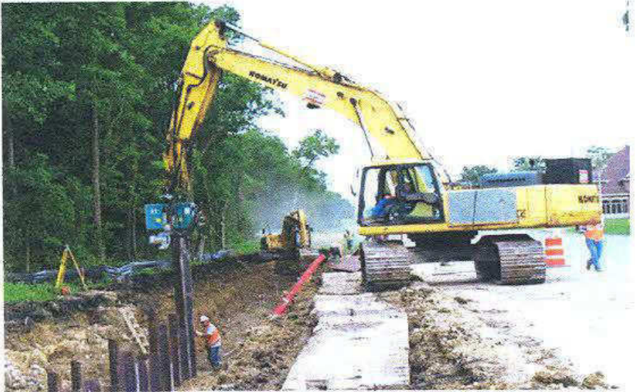
Photo 7.1.3 - 1 Steel sheet pile
