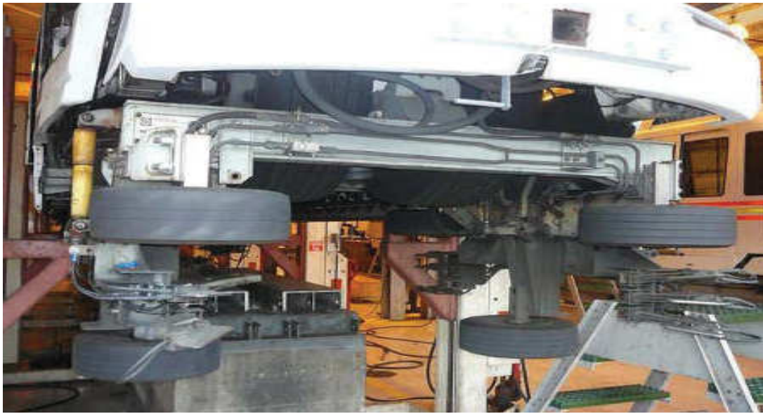
Figure 3.-6-19 Wheel Diagnostic and Tyre Replacement Equipment
