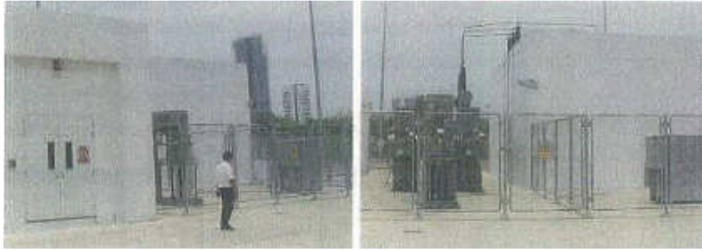
Figure 3.6-22 Typical Bulk Substation
