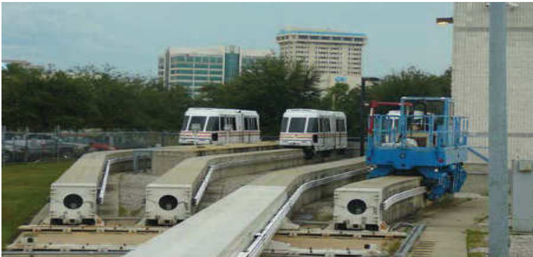
Figure 3.6-23 (b) Stabling Area
