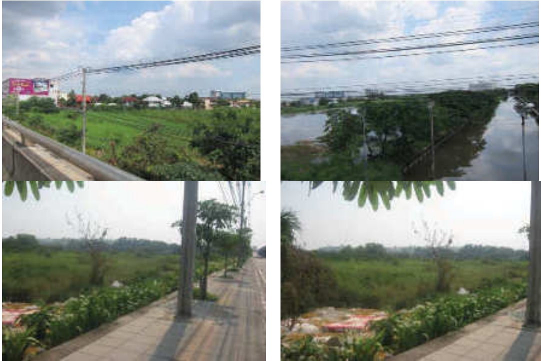
Figure 3.6-2 Existing Conditions of Depot and Park & Ride Building Site at Rom Klao Intersection
