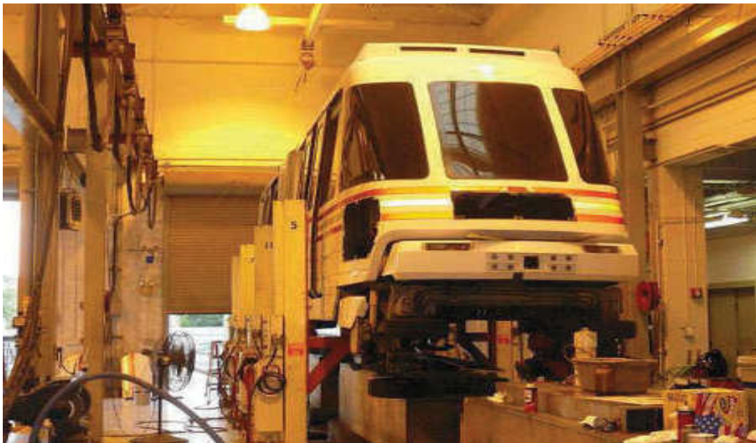
Figure 3.6-20 Internal Conditions of Wheel Diagnostic Facility
