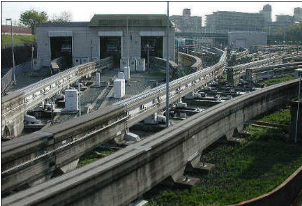
Figure 3.9.3 - 10 Osaka Monorail Depot where has switching of, three, four or five routes
