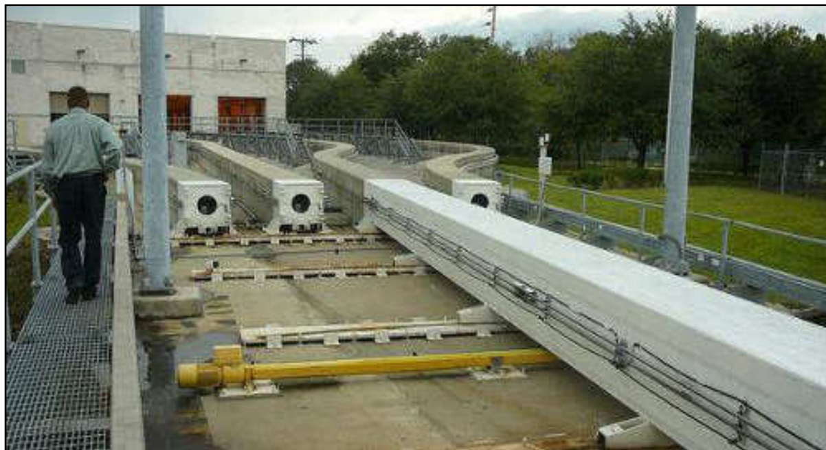
Figure 3.9.3 - 12 The Scenery of Stabling Yard
