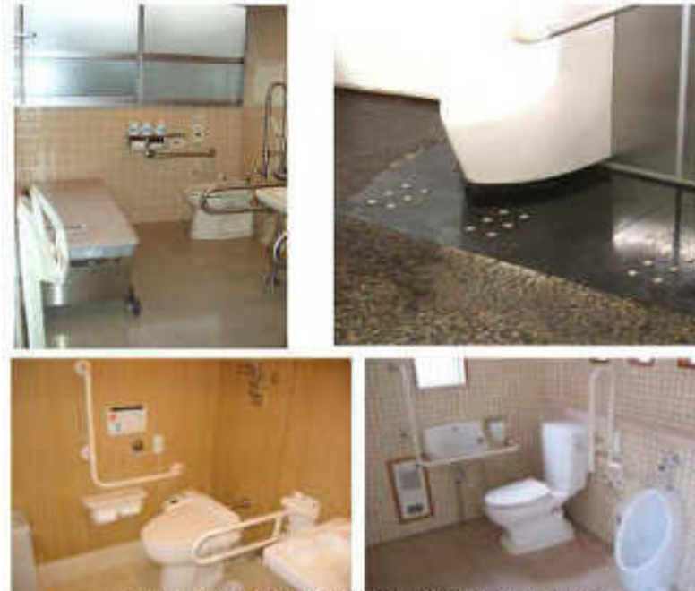
Figure 3.12 - 3 Example of Toilet Designed for the Disabled, Elderly and Pregnant Women
