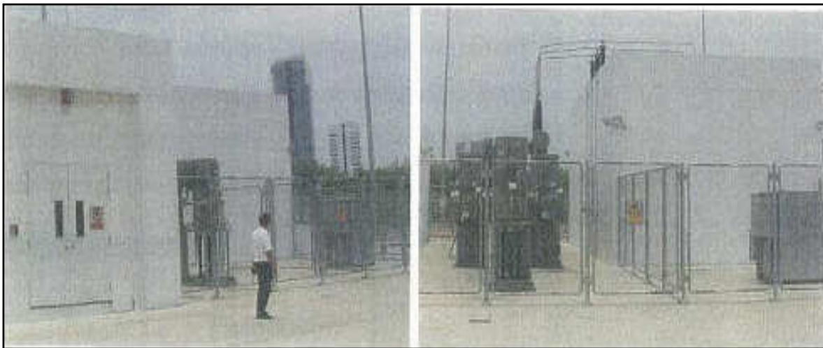
Figure 3.9.3 - 15 Example of Substation Building
