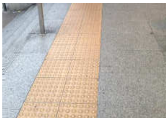
Figure 3.12 - 4 Example of Pathway Designed for the Blind
