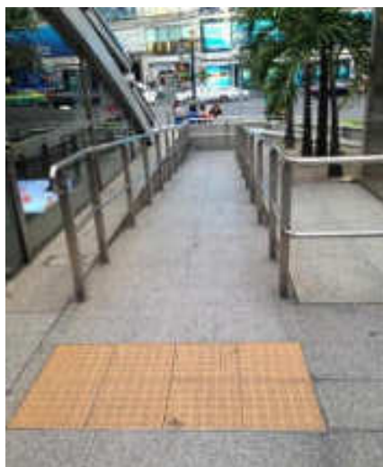
Figure 3.12 - 2 Example of Ramp Designed for Wheelchairs and Elderly
