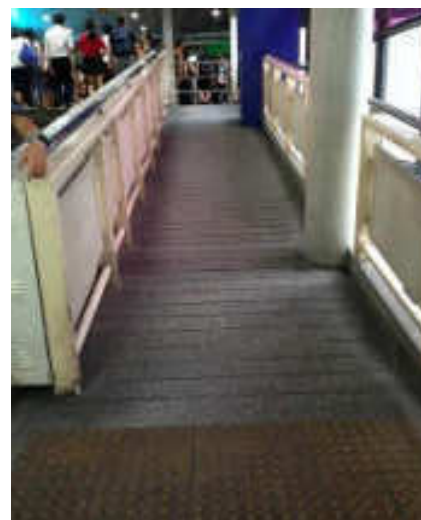
Figure 3.12 - 2 Example of Ramp Designed for Wheelchairs and Elderly
