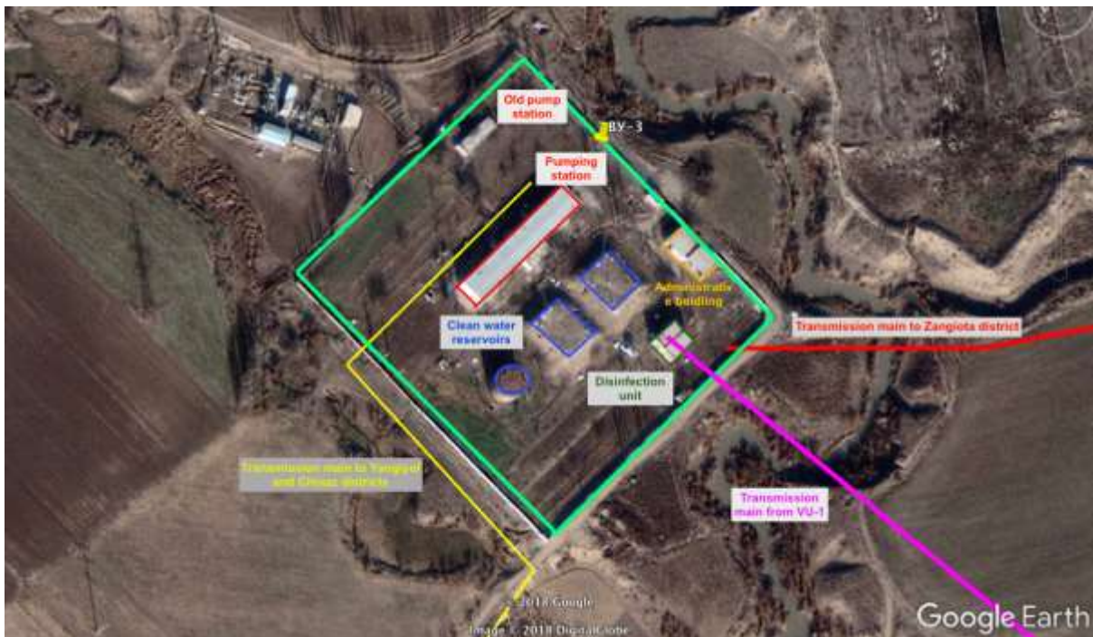
Figure 9: Location of VU-3 and its facilities
