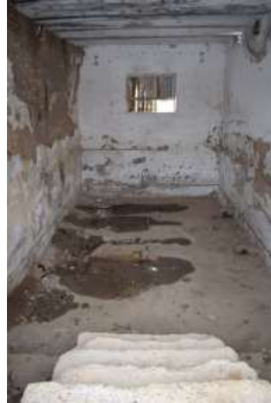
Figure 23: Building of Pump station
