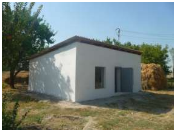
Figure 14: WDC “Khalkabad” – pumping station
