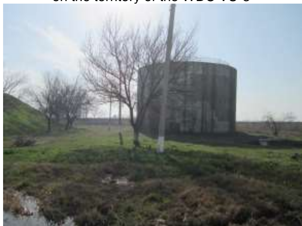
Figure 12: Metal water reservoir
