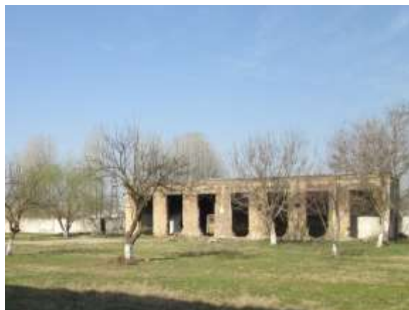
Figure 13: Building of old pump station located on VU-3
