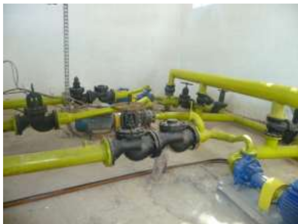
Figure 15: Pump station in WDC “Khalkabad”
