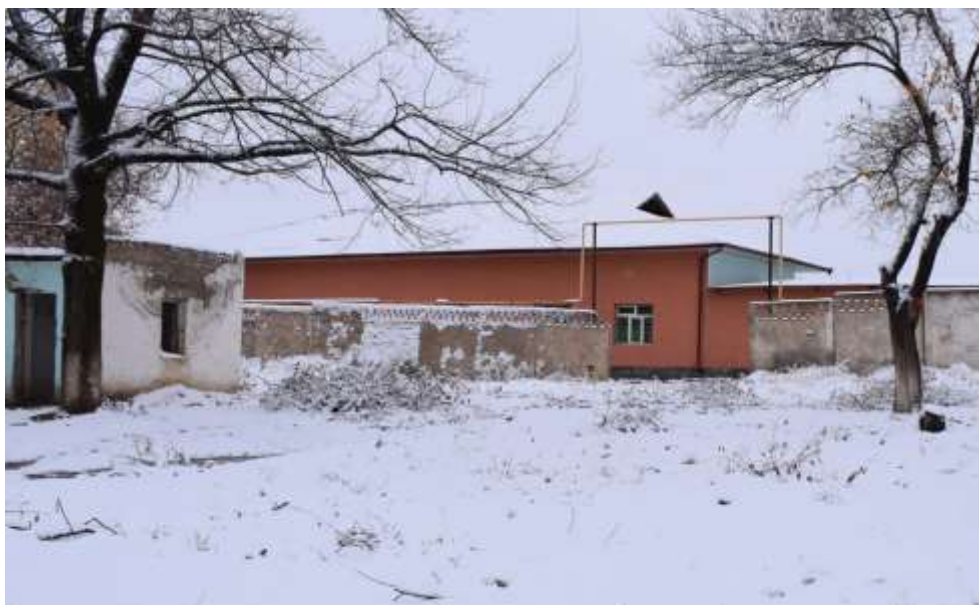
Figure 45: Living houses located next to the Madaniyat WDC
