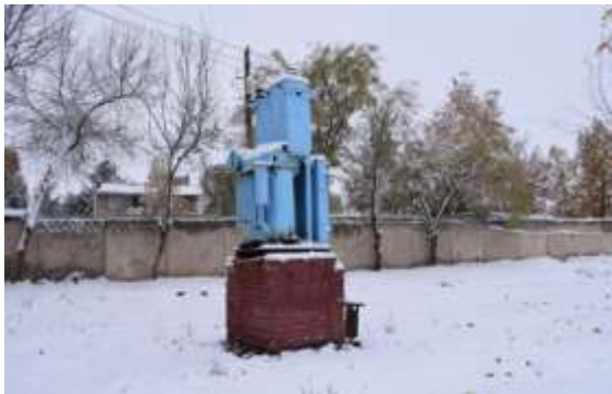
Figure 53: Transformer in WDC “Madaniyat”
