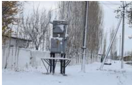
Figure 54: Transformer in WDC
