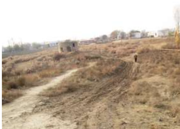
Figure 16: Building of former pump station
