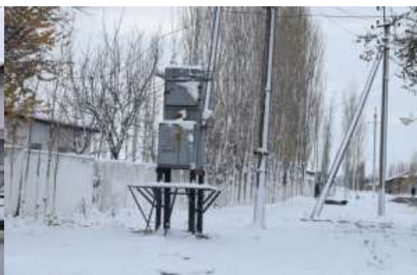
Figure 31: Old transformer on the territory of WDC
