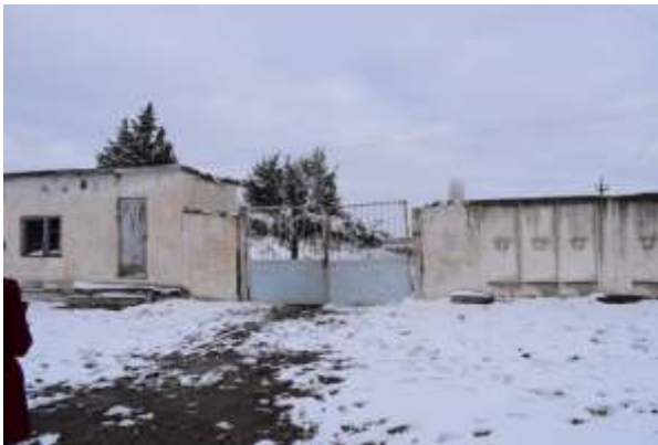
Figure 24: Entrance of WDC "Yangiobod"
