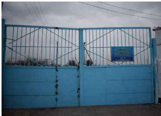
Figure 5: Entrance to VU-1
