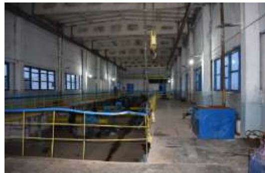
Figure 5a: Pumping station
