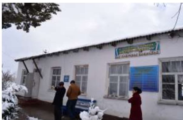
Figure 30: Administrative building of WDC "Chinaz"
