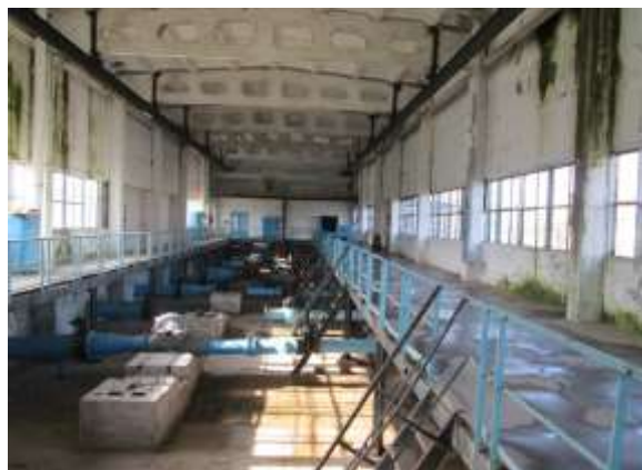
Figure 11: Building of pump station on VU-3
