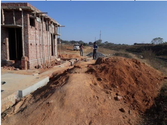
Improper storage of construction material at SP Construction site at CH 467+400 (Nagjua)
