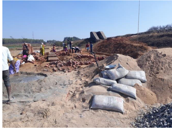
Haphazard storage of construction materials at SSP construction site at CH 448+100
