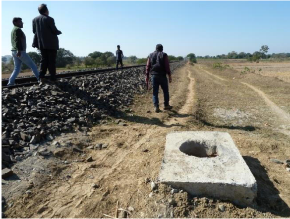
Foundation of Electric Poles left with open hole(unsafe) and no caution tap
