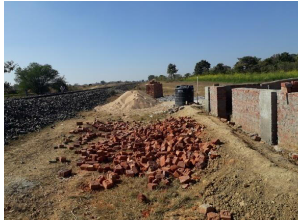
Haphazard storage of construction materials at SSP construction site at CH 448+100
