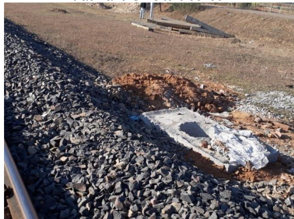
Untidy and unsafe conditions at locations of Electric poles foundation at CH 479+000
