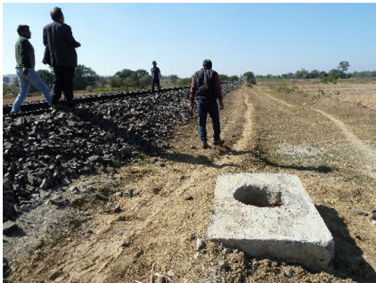
Railway track section near Narkopi Station - Pit for Erecting the Pole Completed - Railway right-of-way free from encumbrance
