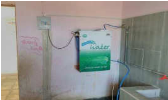
Drinking water facilities in Govt. Primary School
