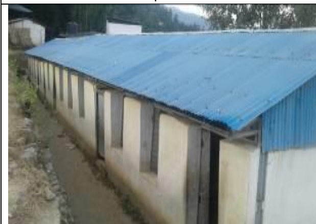
Existing school building
