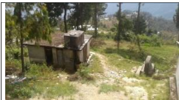
Existing toilet and water supply facilities
