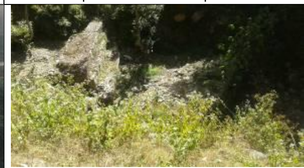
Water stream with gabion wall protection in the south of school compound
