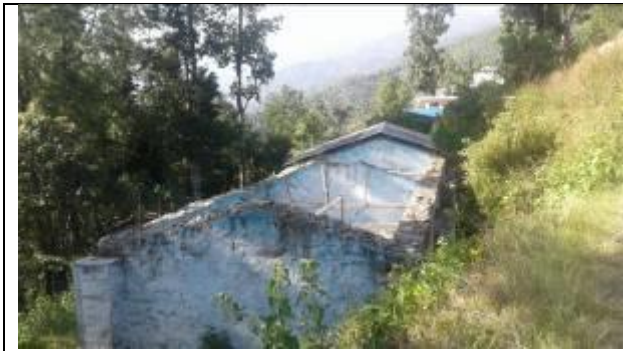
Damaged school building
