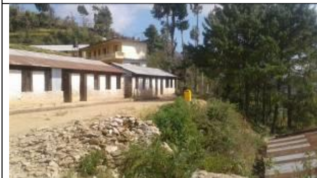
Existing school building
