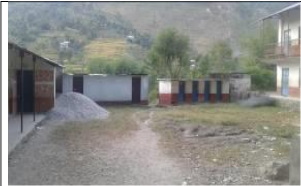
Toilet facilities and construction materials stockpiled
