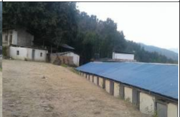
School playground and school buildings
