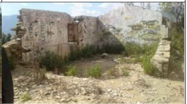
School building damaged by earthquake
