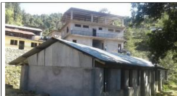
Existing school buildings
