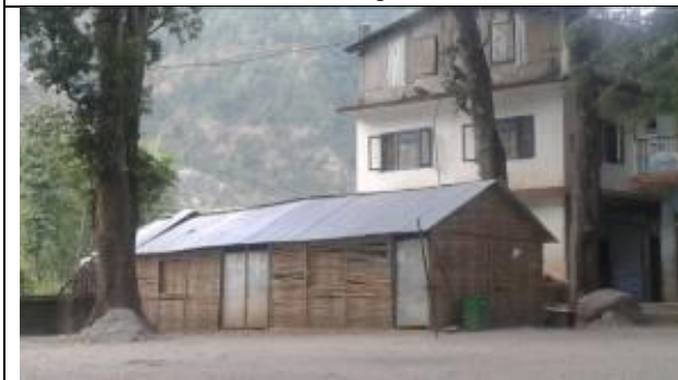
Existing TLC, made by bamboo sheet and CGI sheet
