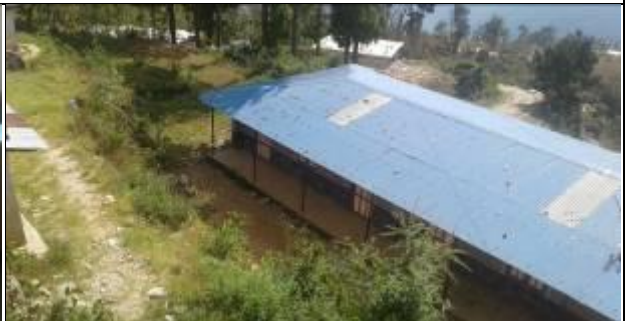
Existing school building
