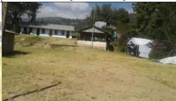
Existing school buildings and playground
