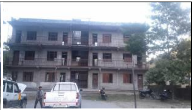
Existing school building
