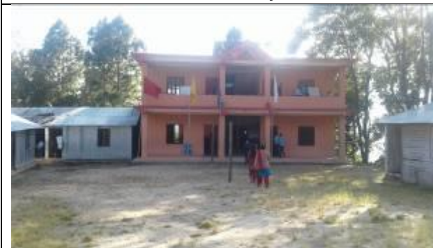
Existing school buildings
