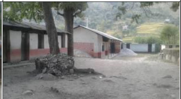
School Buildings and Toilet Facilities
