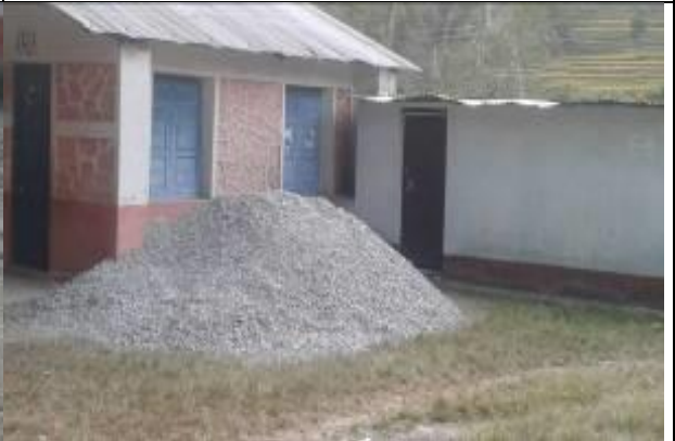
Toilet facilities and construction materials stockpiled
