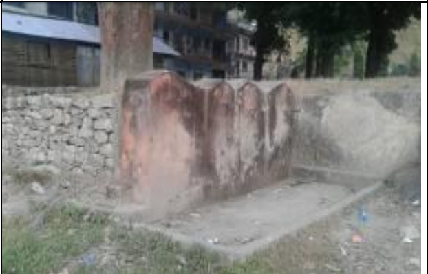
Existing water taps, but not in use
