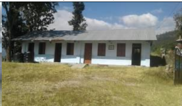
Existing school buildings
