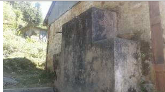
Existing water tap
