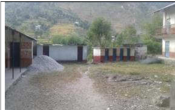
Toilet facilities and construction materials stockpiled
