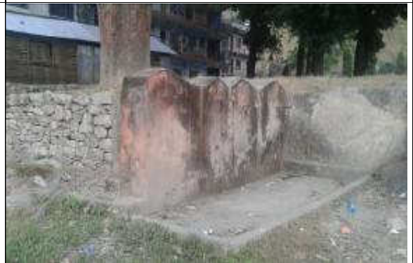
Existing water taps, but not in use
