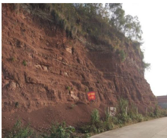
Figure III-26: Current Situation of Bare Hill at Tiangong Hill Area
