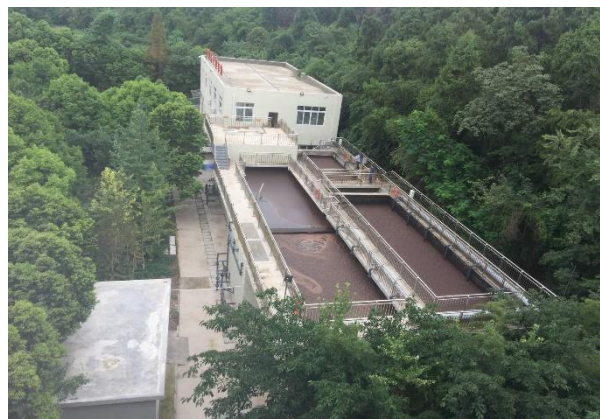
Figure III-20: The Existing Leachate Treatment Facility
