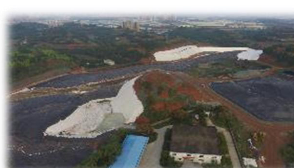
Figure III-22: Existing Landform of Landfill
