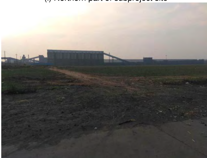
(ii) Western part of subproject site
