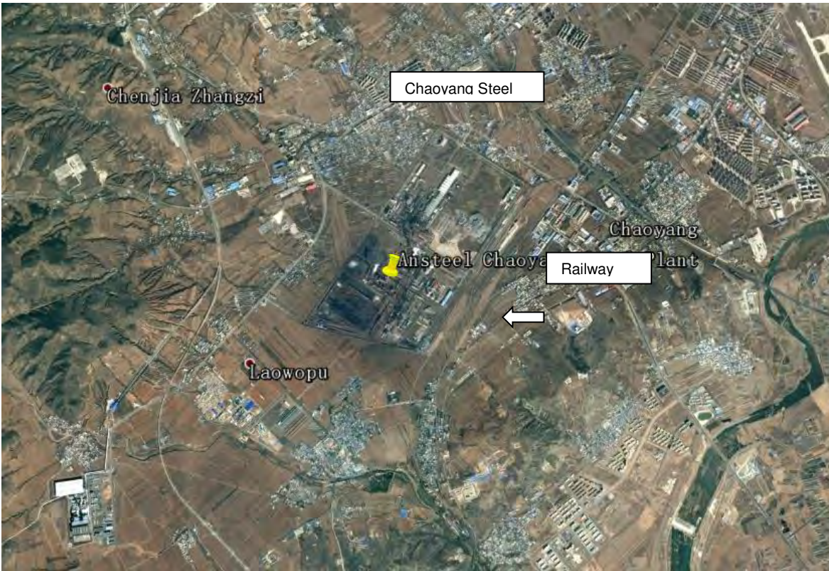
Figure 27: Chaoyang Steel and Surrounding Area
