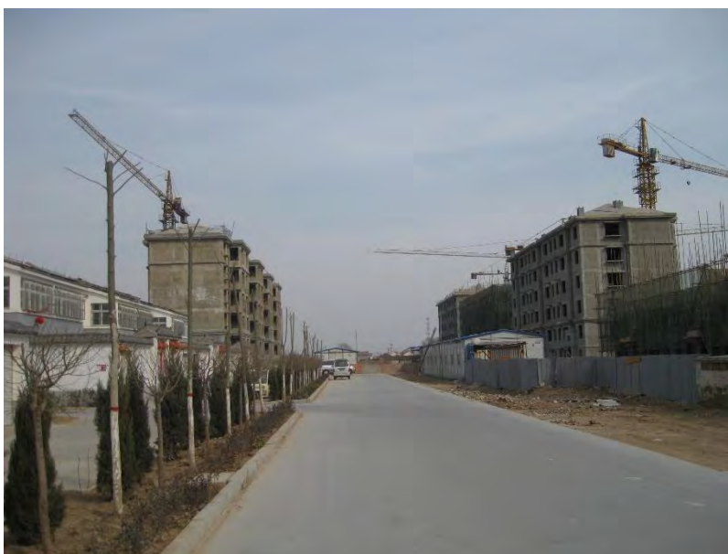
(ii) Road across the subproject site
