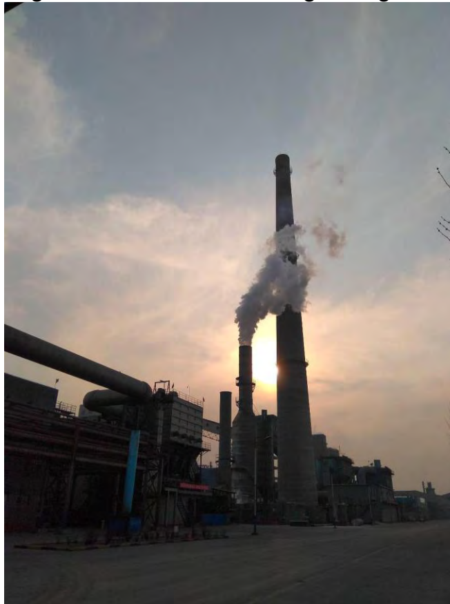
Figure 5: Two stacks of Liheng Coking Plant
