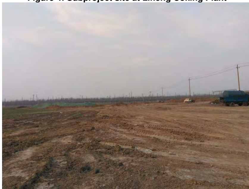
Figure 4: Subproject site at Liheng Coking Plant
