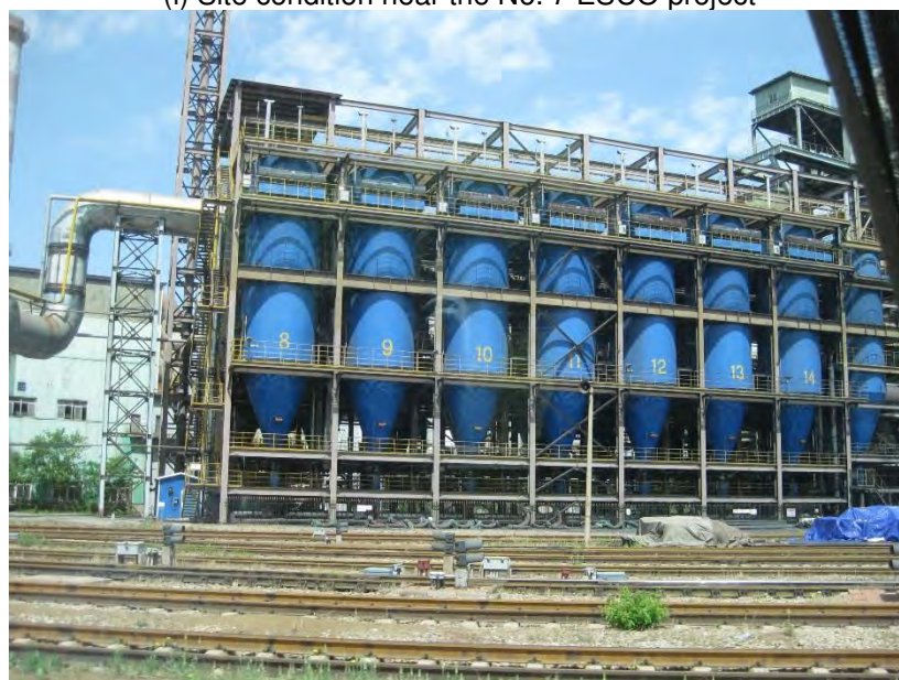
(ii) Site condition near the No. 4 ESCO project
