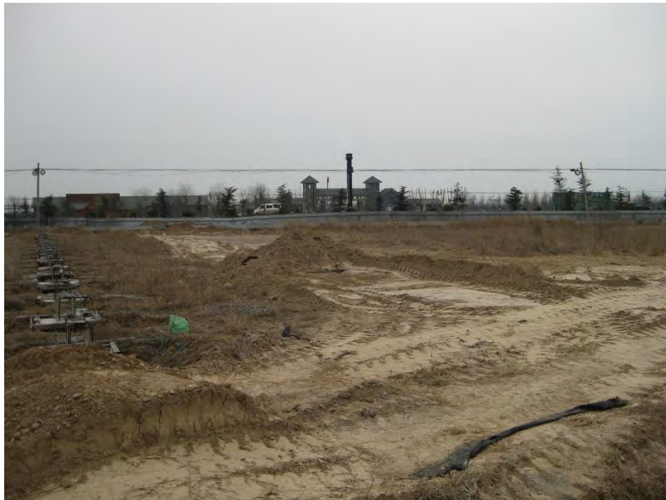
(ii) Western part of subproject site
