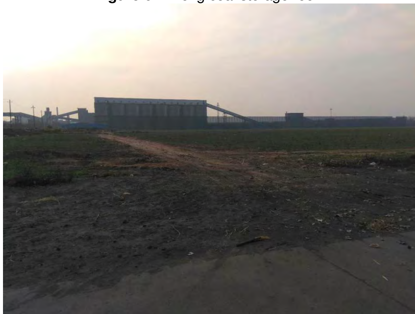
Figure 6: Liheng coal storage room
