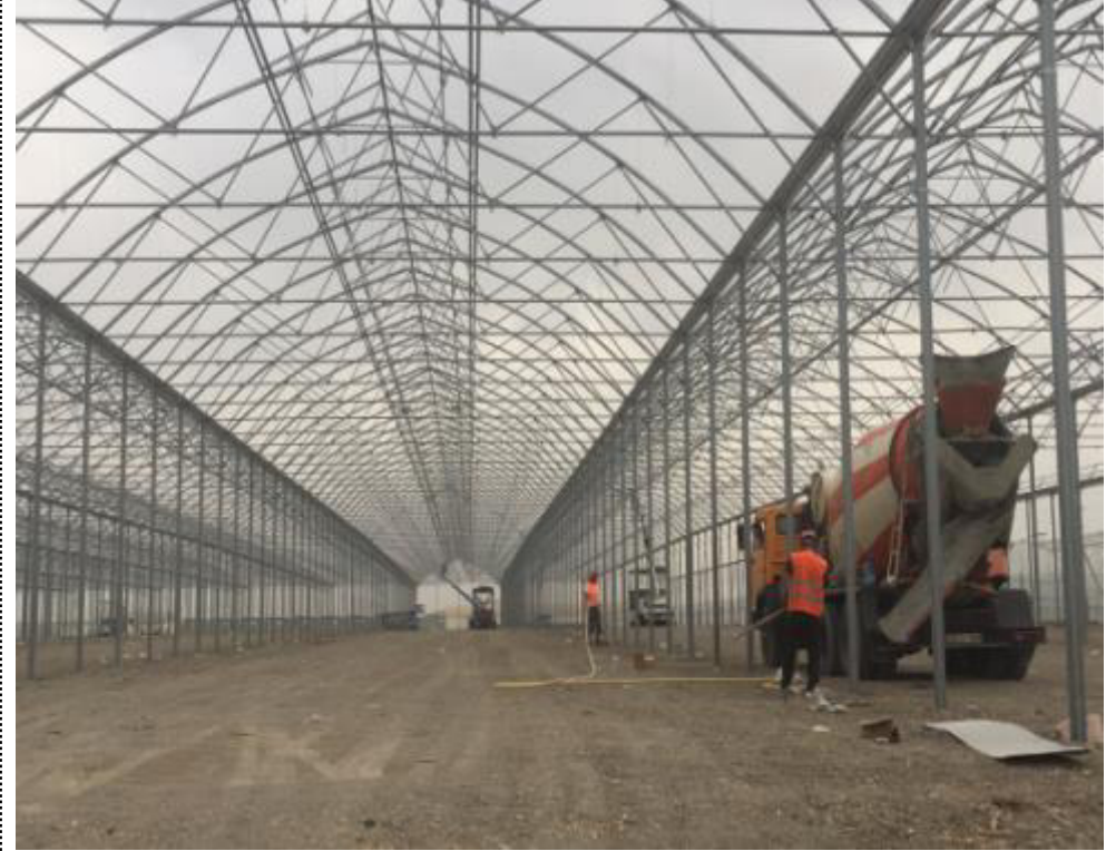
Photo10: Ongoing construction site activities
