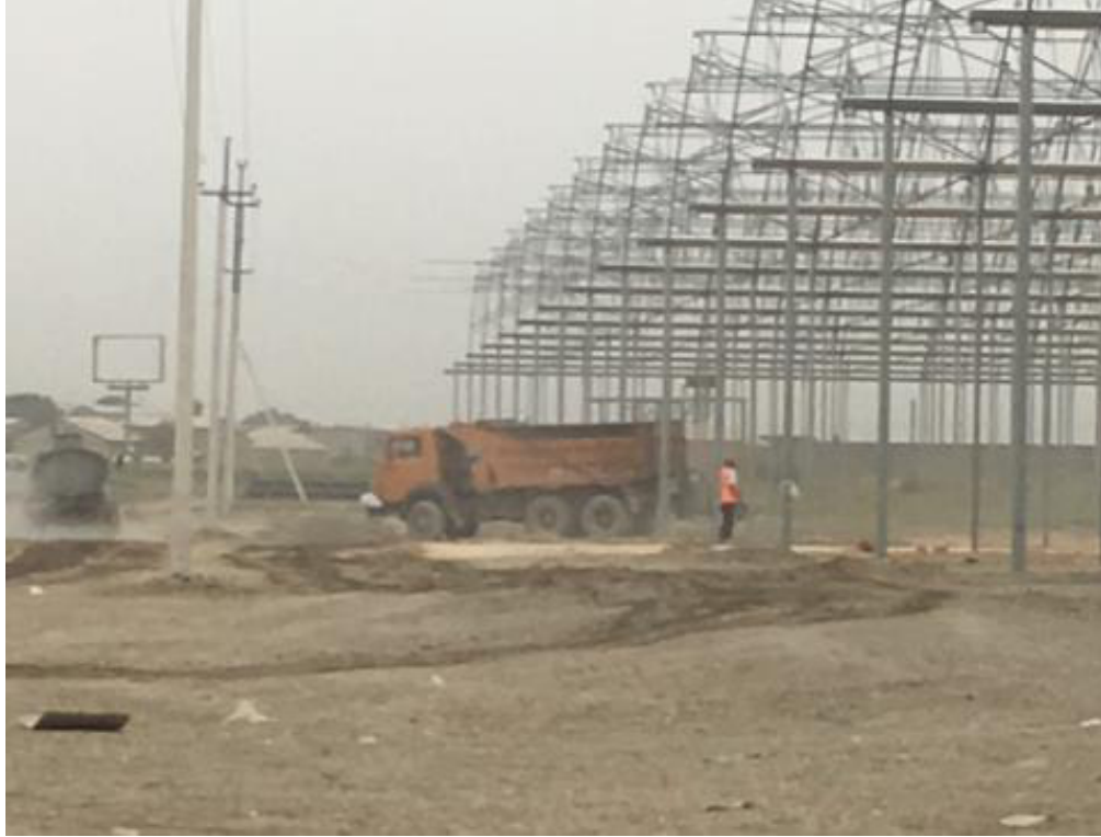
Photo 9: Ongoing construction site activities
