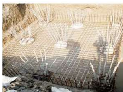
pile cap reinforcement
