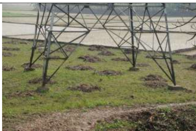
Plate 28 TL tower footing, 132 kV, in a paddy field
