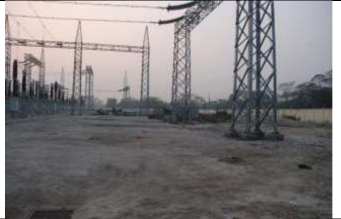
Plate 20 An area set aside for the GIS bays- Barisal GSS
