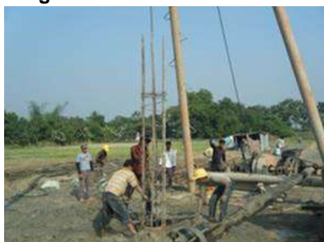
placing of steel ring bunds
