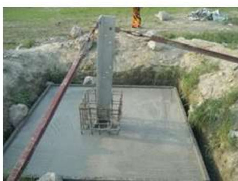
Casting CC into tower foundation
