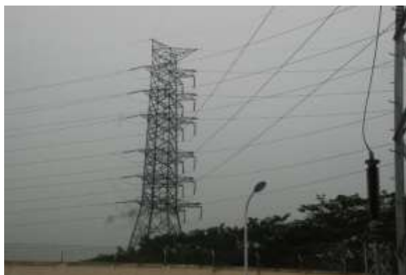
Picture 4. Double Circuit line-in line-out terminal tower
