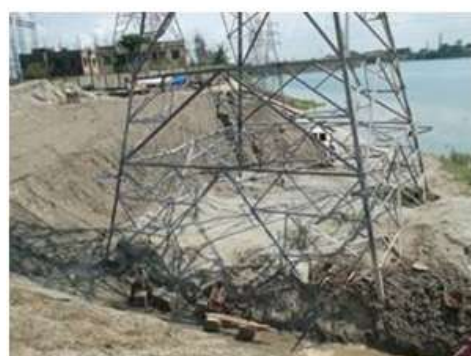
Placing tower on its foundation
