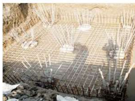
pile cap reinforcement
