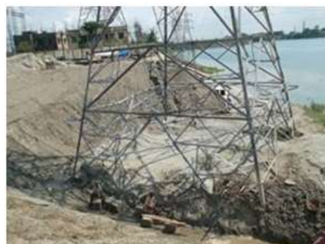
Placing tower on its foundation
