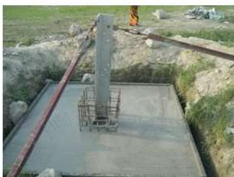
Casting CC into tower foundation
