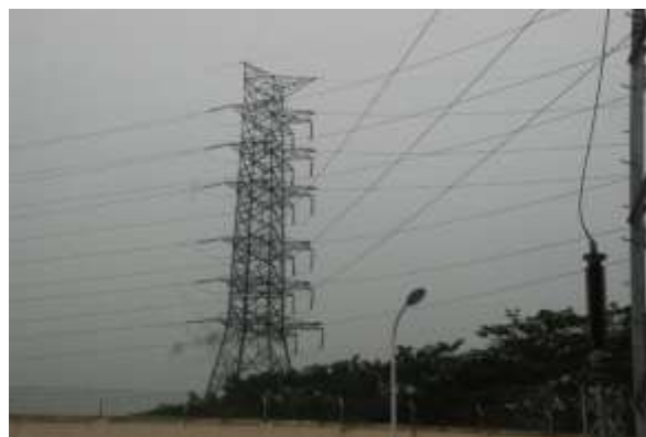
Picture 4. Double Circuit line-in line-out terminal tower
