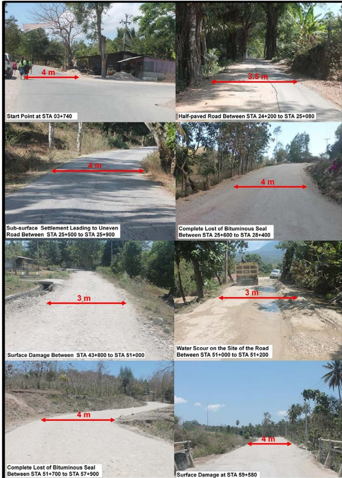
Figure 4.5: Typical road conditions
