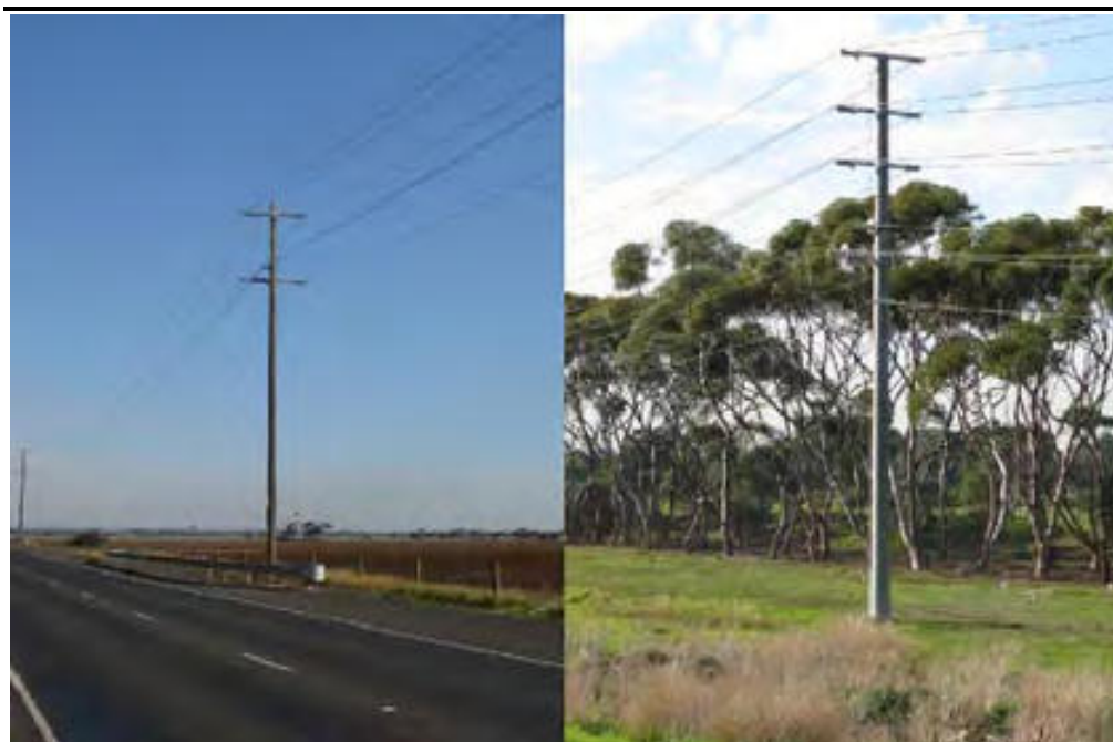
Figure 3.9 (Left to right) Single Circuit 66 kV with Subsidiary (Wood poles), Double Circuit 66 kV with Subsidiary
