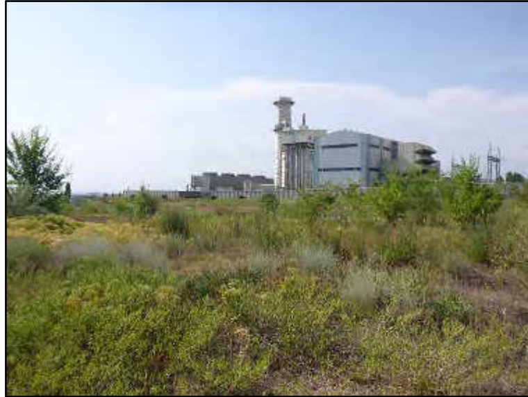
Figure 6-1: Typical vegetation at the construction site (YCCPP-1 in background)
