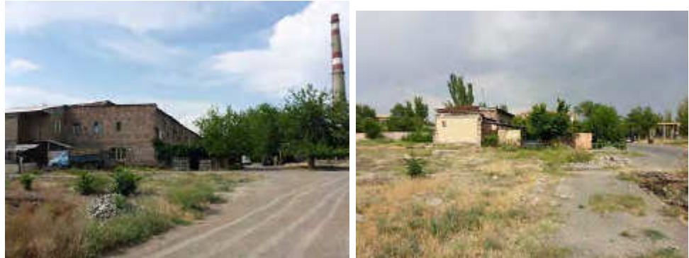
Figure 6-7: Illegal houses located northeast of YCCPP-1 and YCCPP-2
