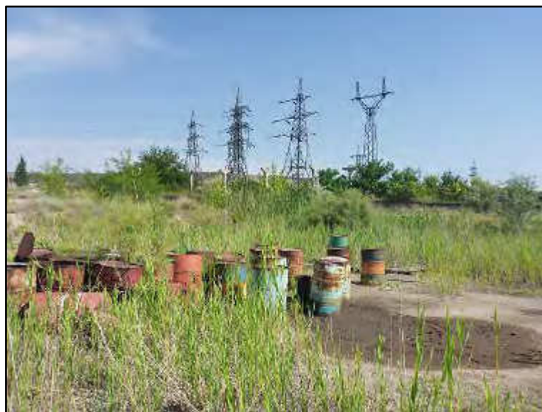
Figure 6-2: Oil leakage near to some empty oil drums at YCCPP-2 site
