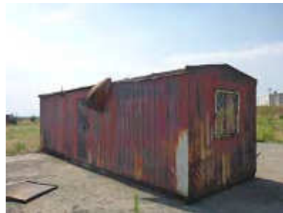
Figure 7-3: Metal cabin on concreted area
