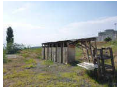
Figure 6-5: Old toilets and wash basins
