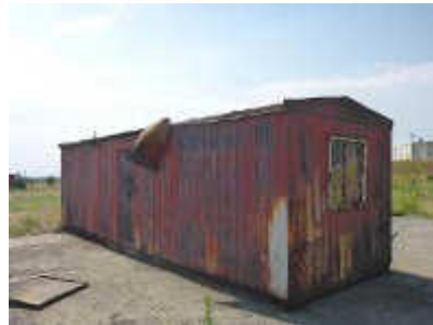
Figure 6-4: Metal cabin on concreted area
