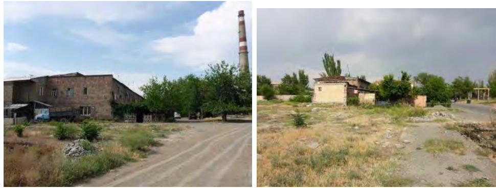
Figure 5-13: Illegal houses located northeast of YCCPP-1 and YCCPP-2 (Source: Fichtner, July 2017)
