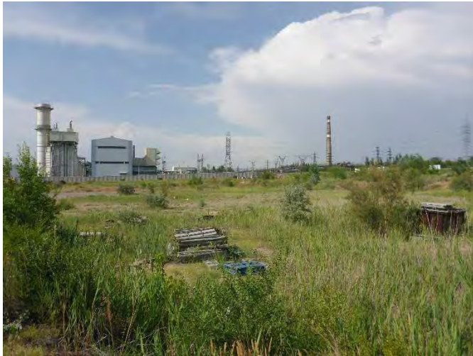
Foto 7: On the site, view to N with TPP1
