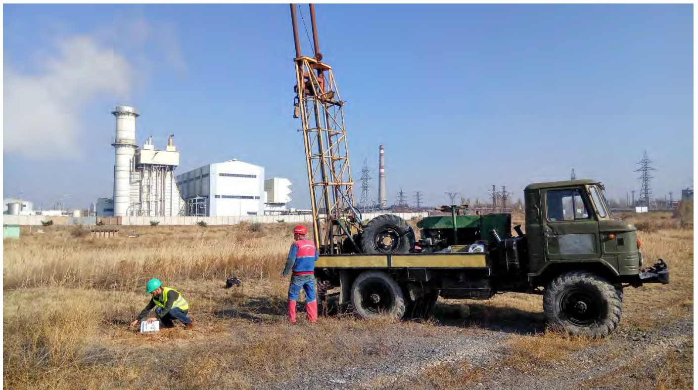
Foto 9: Drilling works from November, 15 th of borehole 14 (4 meters)
