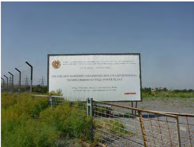
Foto 1: Entrance area to YTPP-2 site
