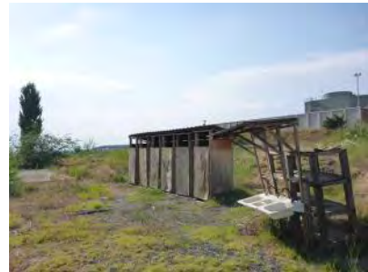
Figure 6-5: Old toilets and wash basins
