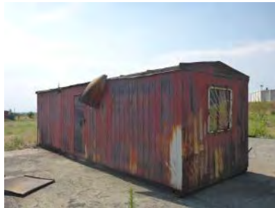
Figure 6-4: Metal cabin on concreted area
