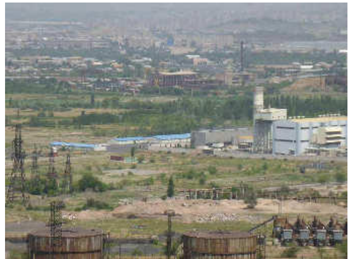
Foto 2: Area overview with construction site (center) and TPP-1 on the right side
