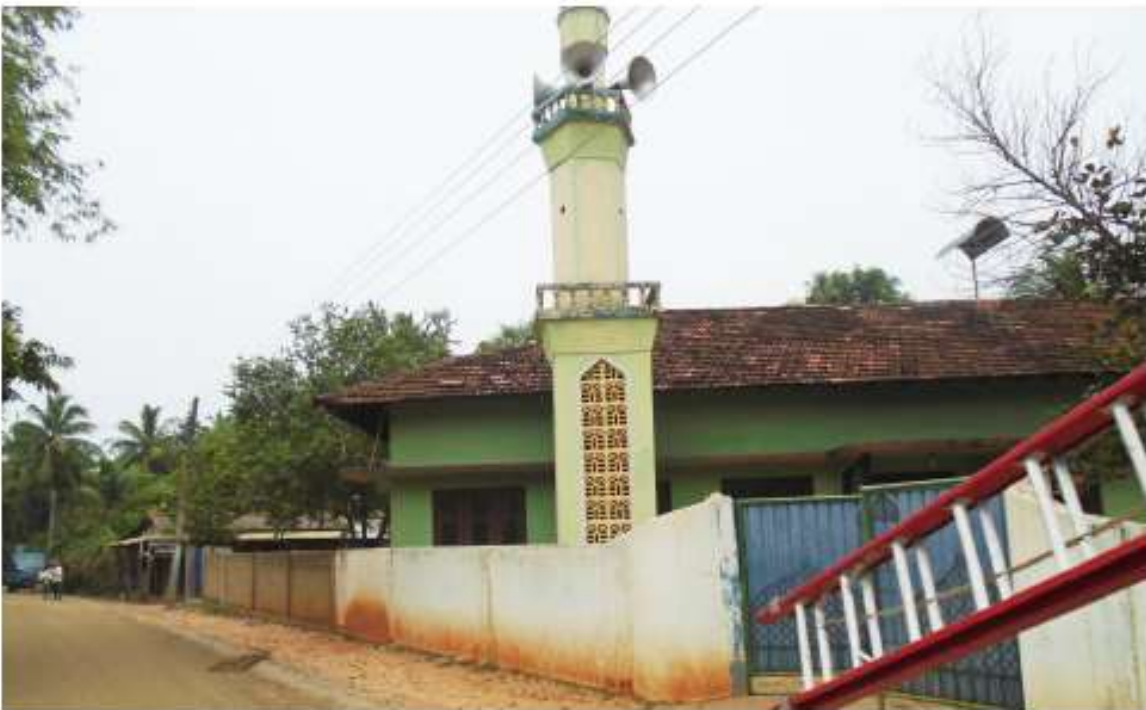
Mosque located at 0.460km RHS of the road
