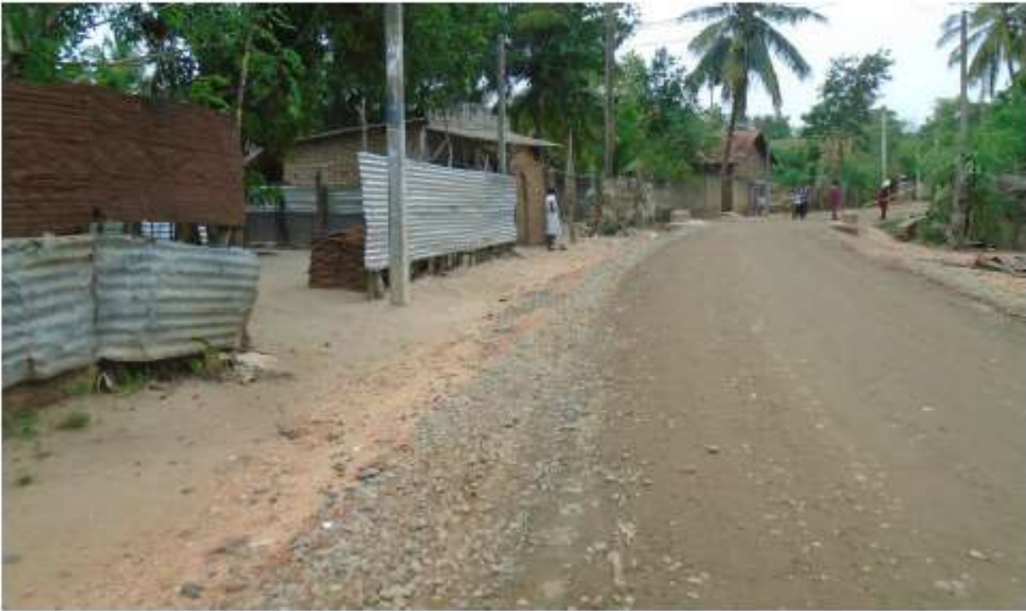
The road is under upgrading work.
