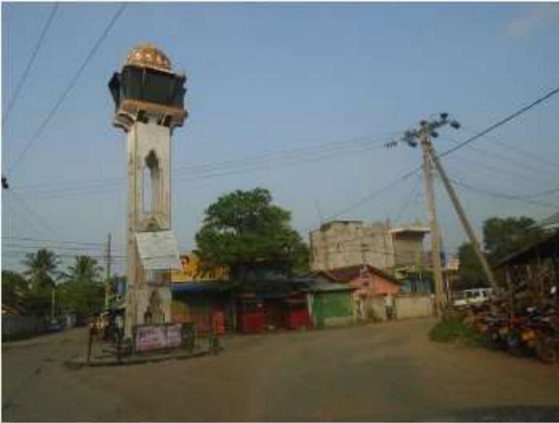
Figure 3: Clock tower located at 0,900km
