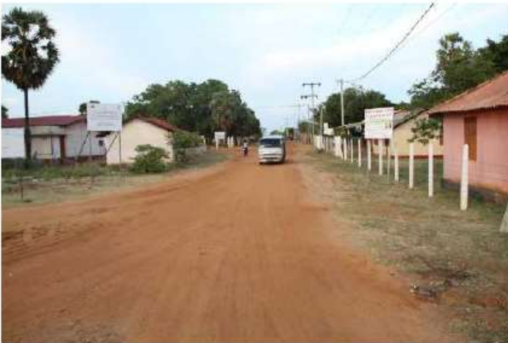
Road condition at the 0+400km+.
