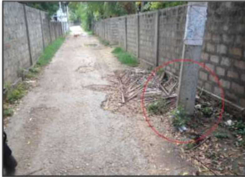
Figure 7: An electricity pole with in ROW - St Xavier Sea side Road Section II-Alvai North GN division-Point Pedro DS division-Jaffna- 100m
