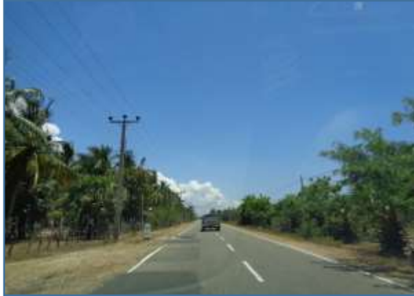
Existing condition of ROW at ch. 50+000 (near end point ch. 108+000)
