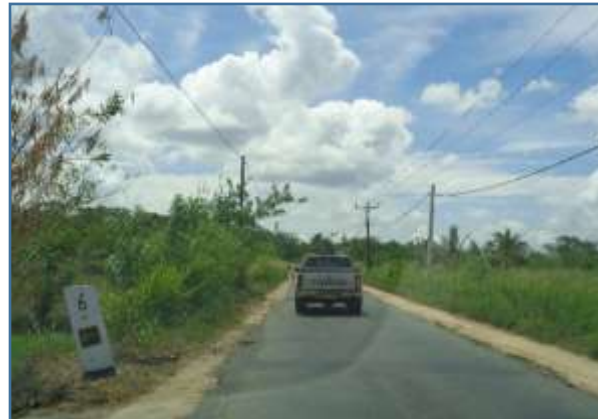
Existing road, ROW condition at ch. 6+000
