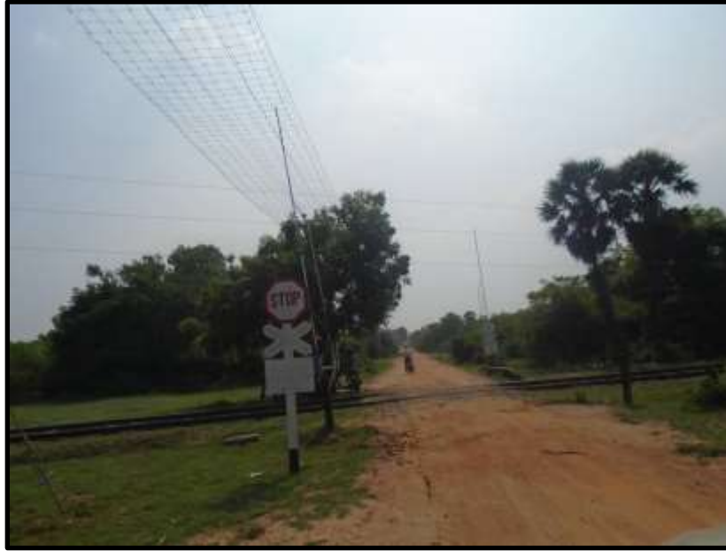
Figure 16: Potthanai Road crossed by railway line- Koralai Pattu South (Kiran) DSD - Batticaloa district
