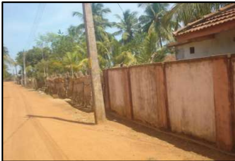
Figure 6: An electricity pole with in ROW - Vaikal Kulathu Road sec. i - Manmunai South-West DSD - Batticaloa district- 0+100 m.
