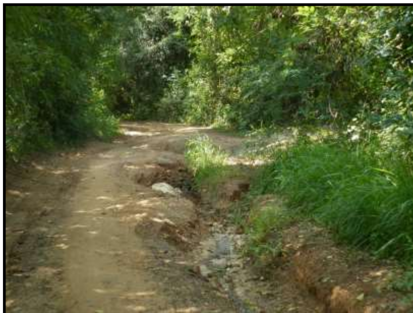
Figure 12:.. Soil erosion in road section due to run off water - From Bodagolla MV Sangadasa's house to Ambagahawella Sec .I -Ampara DSD- Ampara district-0+900 m
