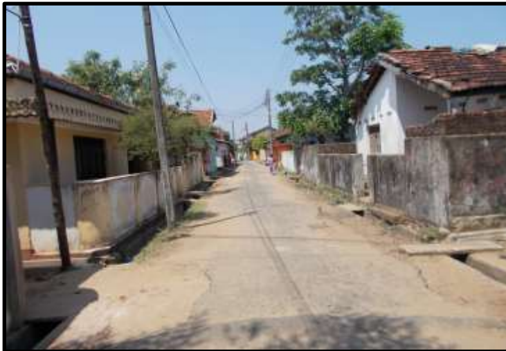
Figure 8: An electricity pole with in ROW - Mawadichenai Road - Verugal/ Echchilampattai DSD - Trincomalee district- 0+50 m.
