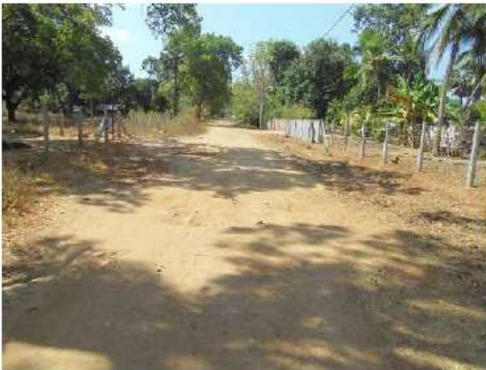
Roadside environment at 0+200-0+300km
