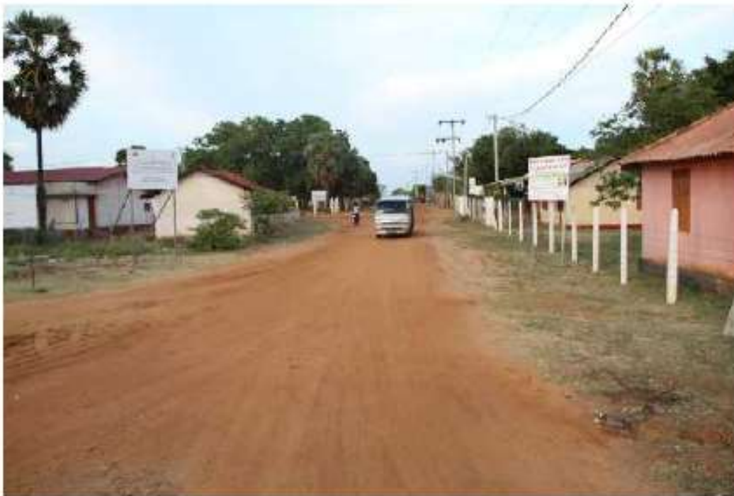
Road condition at the 0+400km+.
