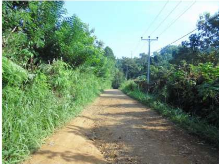
Road surface and roadside environment at 2+500-2+600km
