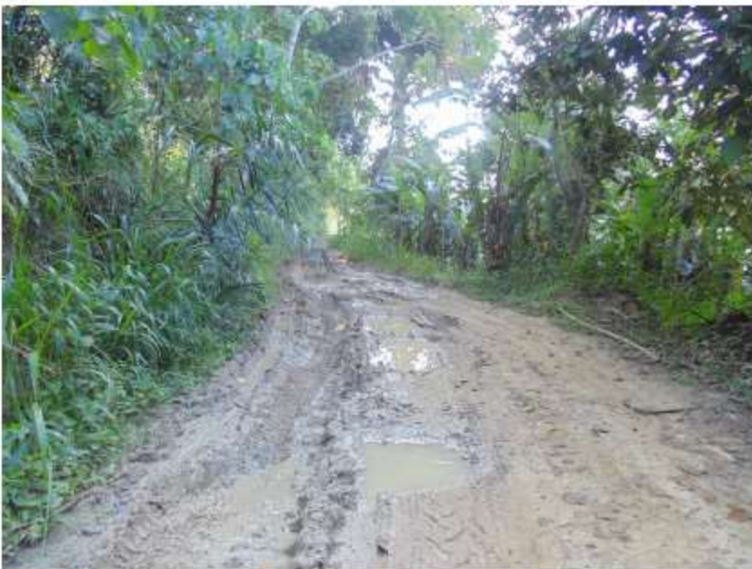
Muddy surface and roadside environment at 0+000-0+100km
