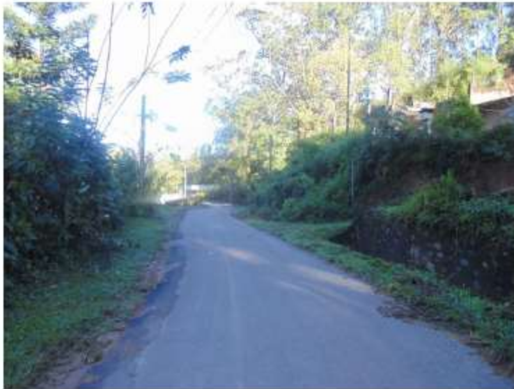
Existing ROW and the carriageway at 0+400-0+500km
