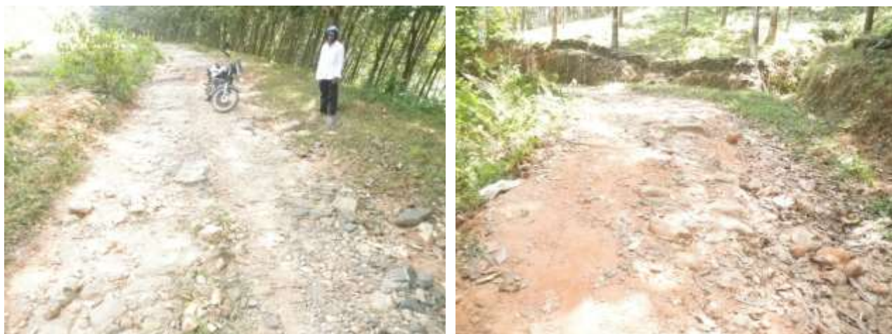
Figure 7: Location where Nadraj lost his life due to poor road condition
