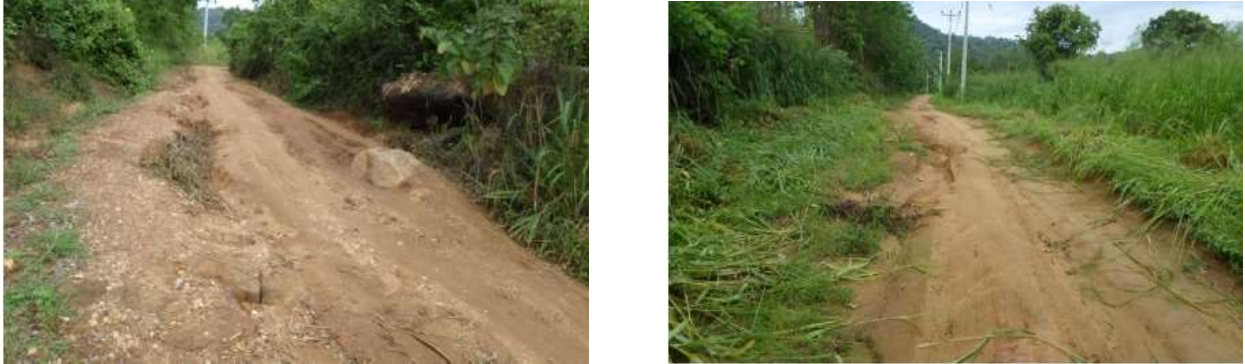
Figure 6: Existing Road Condition
