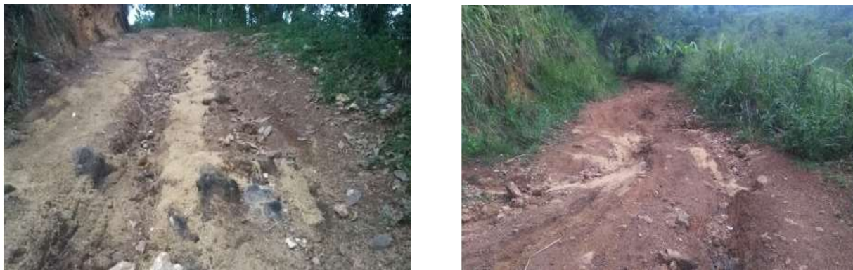
Figure 5: Existing Road Condition
