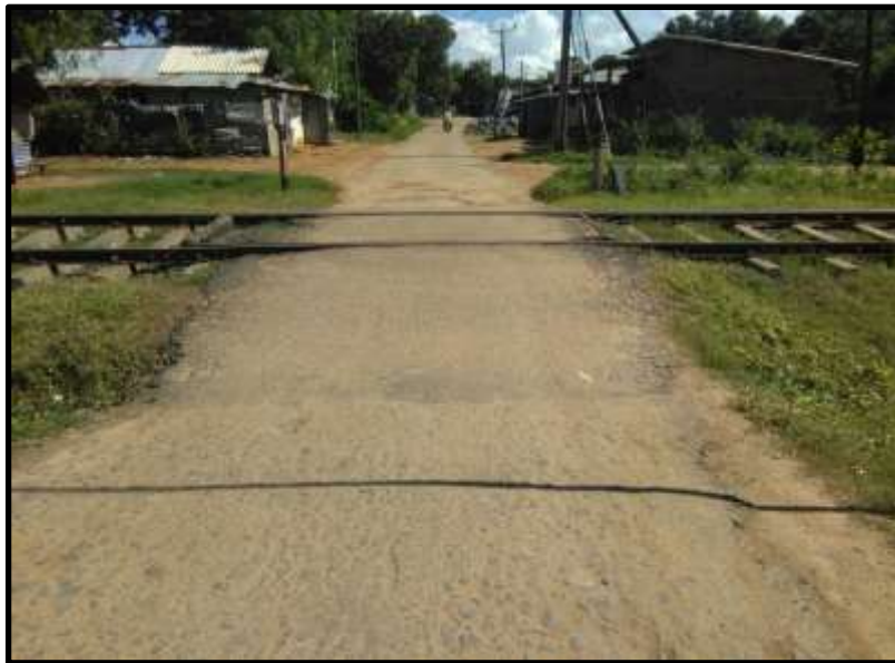
Figure 15: Shiraj Nager Main Road crossed by railway line- Thambalagamuwa DSD - Trincomalee district
