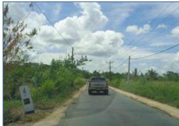
Existing road, ROW condition at ch. 6+000
