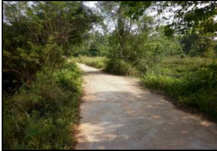
Figure 4: Over grown vegetation- Dambadeniya school road (concrete road) - Mahaoya DSD-Ampara district-0+600m
