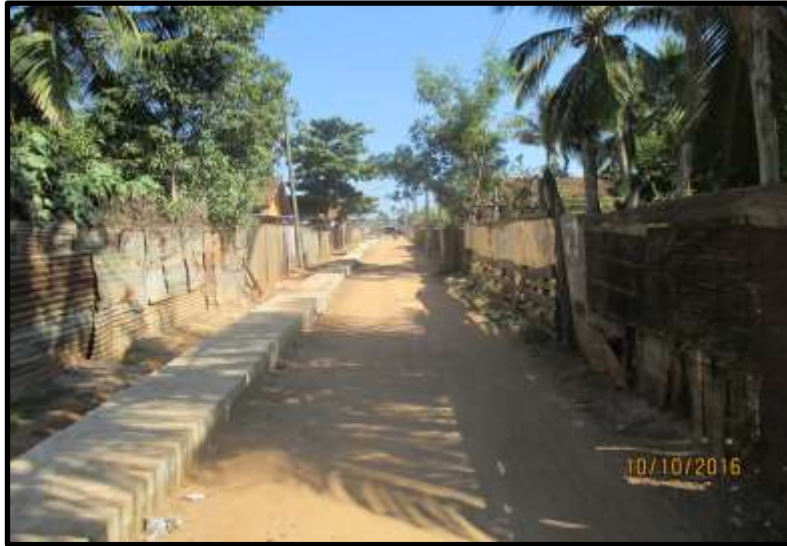
Figure 5: A drainage channel with in ROW - Ahamod Hirashi Road, Semmanodai Road, Koralai Pattu Central DSD --Batticaloa district
