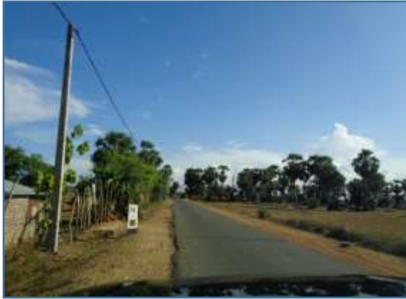
Existing condition of ROW at ch. 14+000
