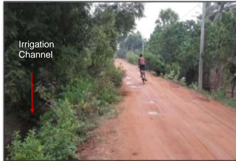
Figure 10: A Small irrigation canal is located close to a road section- Sulipuram Nelliyan Road- Jaffna District
