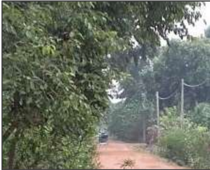
Figure 4: Over grown vegetation- Sulipuram Nelliyan Road- Jaffna District
