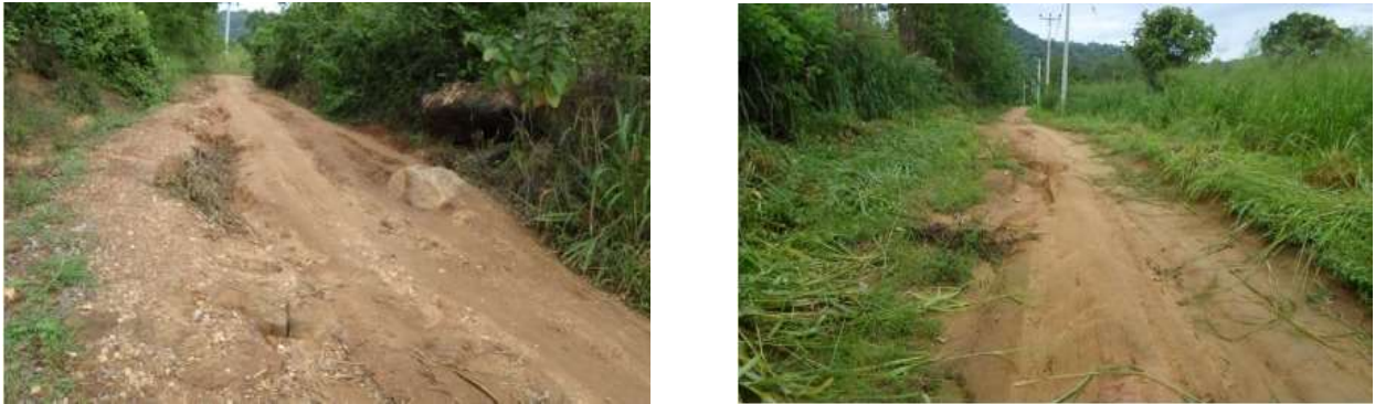
Figure 6: Existing Road Condition
