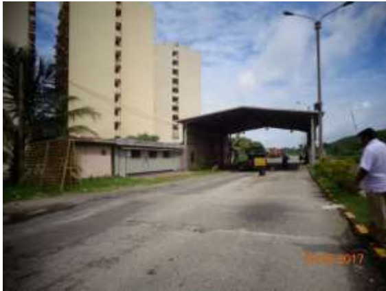
Opening Gate at Ingurukade Junction-Ch- 0+140
