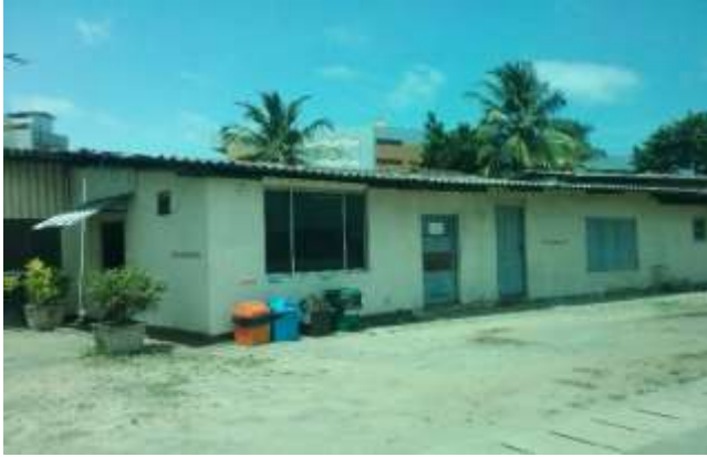
Rest Rooms for Workers. -Ch- 3+400 – 3+800
