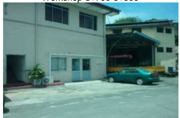
Stores building Ch 3+700-3+900
