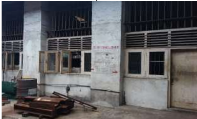
Workshop Building. - Ch 3+700-3+900
