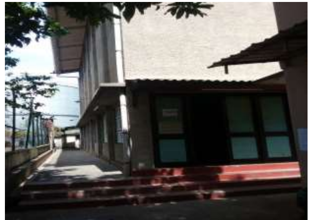
SLPA Indoor Stadium- Ch 1+700-1+800
