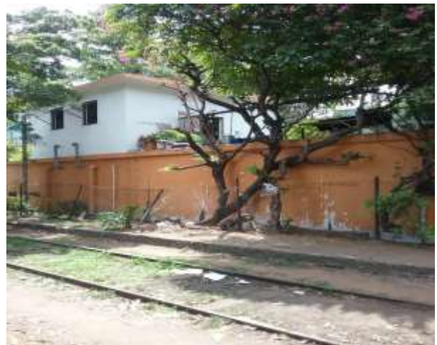
Parapet Wall and Railway Line to be shifted. Ch-2+400 to 3+500
