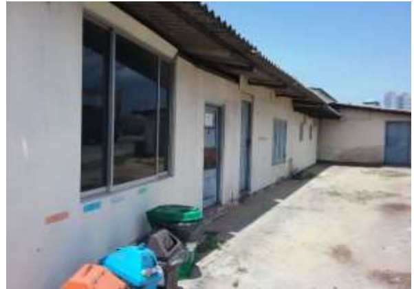
Stores room from ch 3+500 – 3+600
