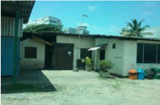
Store room ch 3+500 – 3 + 600
