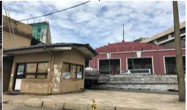
Rest Room Ch 3+700-3+900
