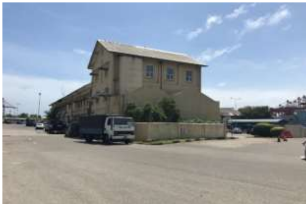
Partially demolishing building. Ch- 4+600-4+900
