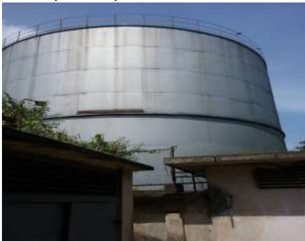
Oil Tanks to be pruned (Removing of two Rings)
