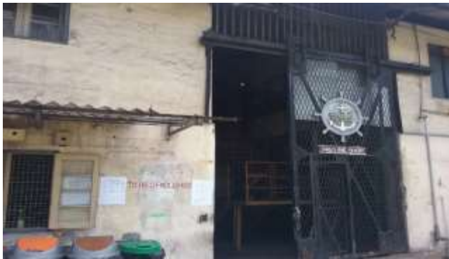
Machine Workshop- Ch 3+700-3+900
