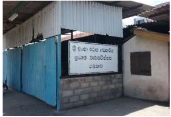
Store rooms Ch 3+500 – 3 +600
