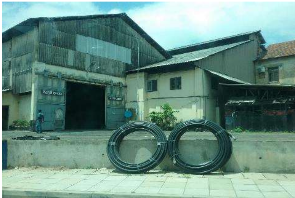
Photograph No.09 – Main Store Complex Ch- 3+573
