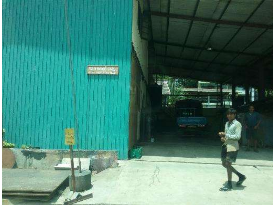
Photograph No.08 Fabrication Workshop- Ch 3+532
