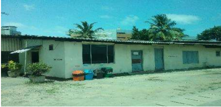
Photograph No.05 – Work Shop Ch- 3+457
