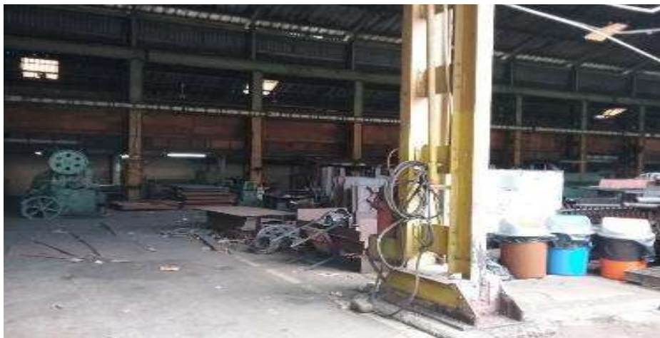
Photograph No.11.a- Inside of the Workshop- Ch 3+652
