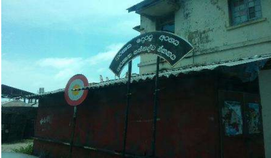
Photograph No. 10- Rest Room / Security Section Building- Ch- 3+659
