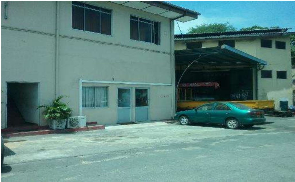
Photograph No.13- Stores/ Welfare Building Ch 3+673
