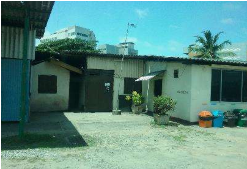
Photograph No.06 Work Shop Ch-3+497
