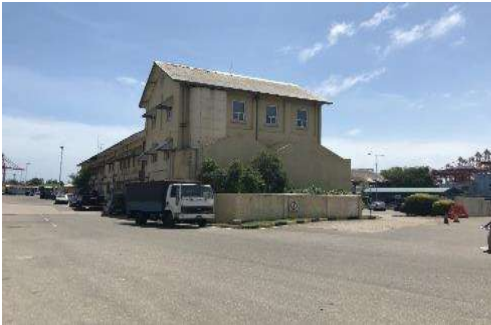
Photograph No.15 – Chairman's Office Ch-4+900
