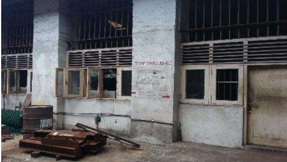
Photograph No.12 - Workshop Building. – Ch- 3+700
