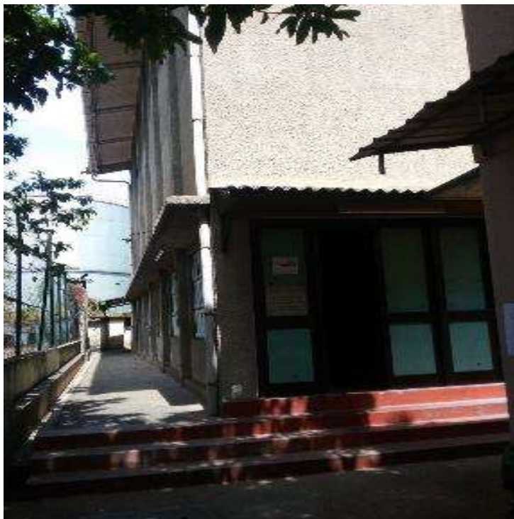
Photograph No. 03 – Indoor Stadium Ch -1+735
