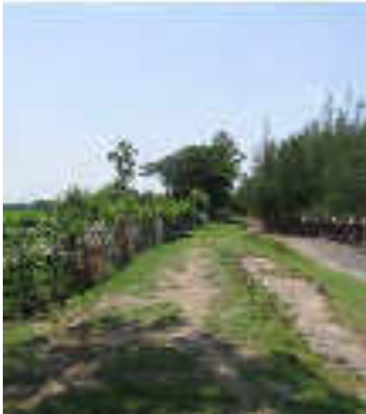
Beribandh – Coastal Embankment
