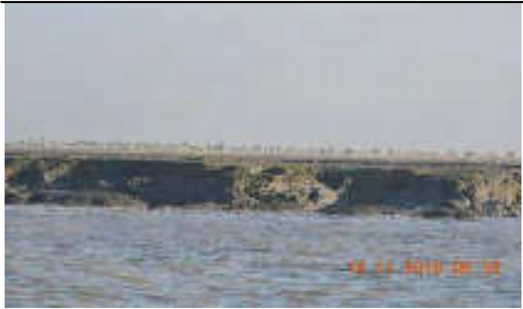
Erosion at Southern Bank near Tabaleshwar
